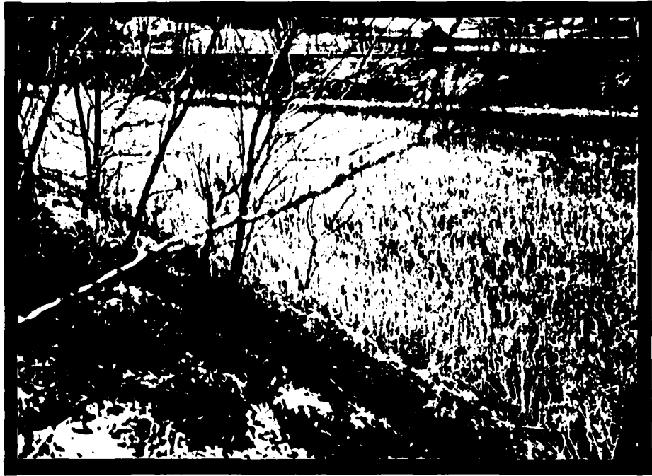
Photo 3 Downstream Toe Area showing extreme swampy condition along central portion of toe.
