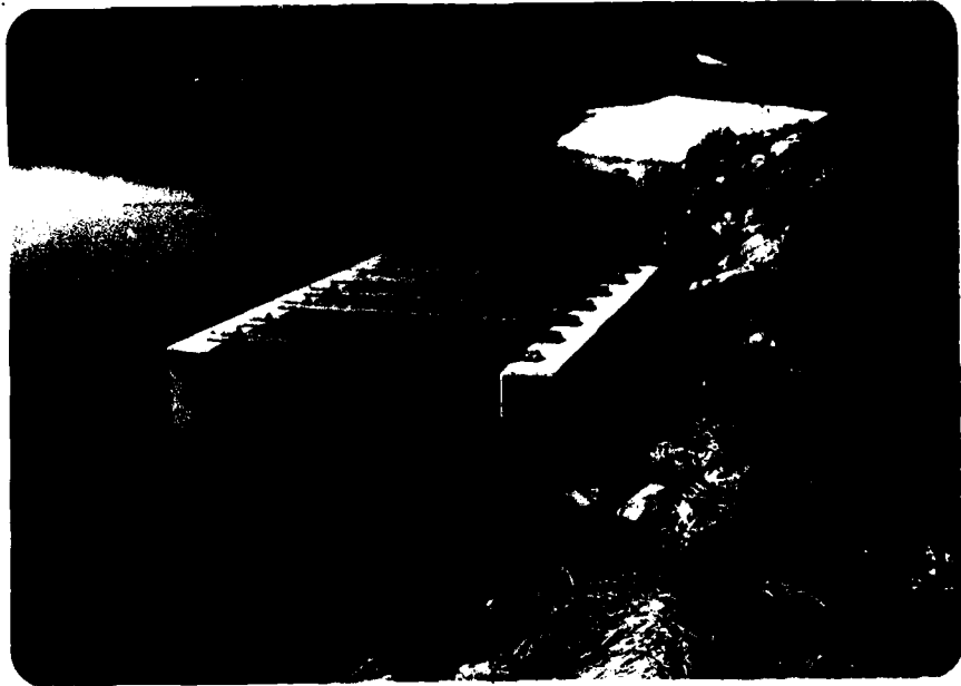
7. CONCRETE INTAKE STRUCTURE FOR SERVICE SPILLWAY. NOTE TRASH RACK.
