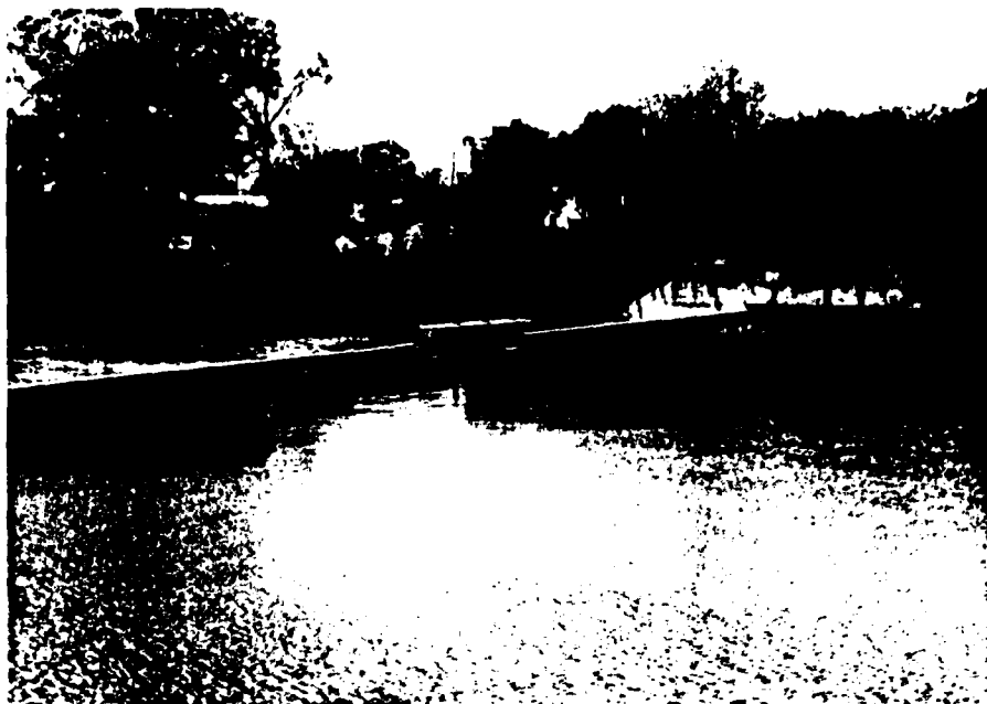
C. Upstream side of dam
