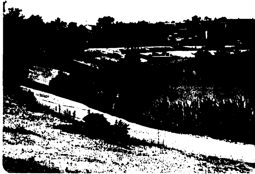
A. Upstream slope of dam and asphalt slope protection
