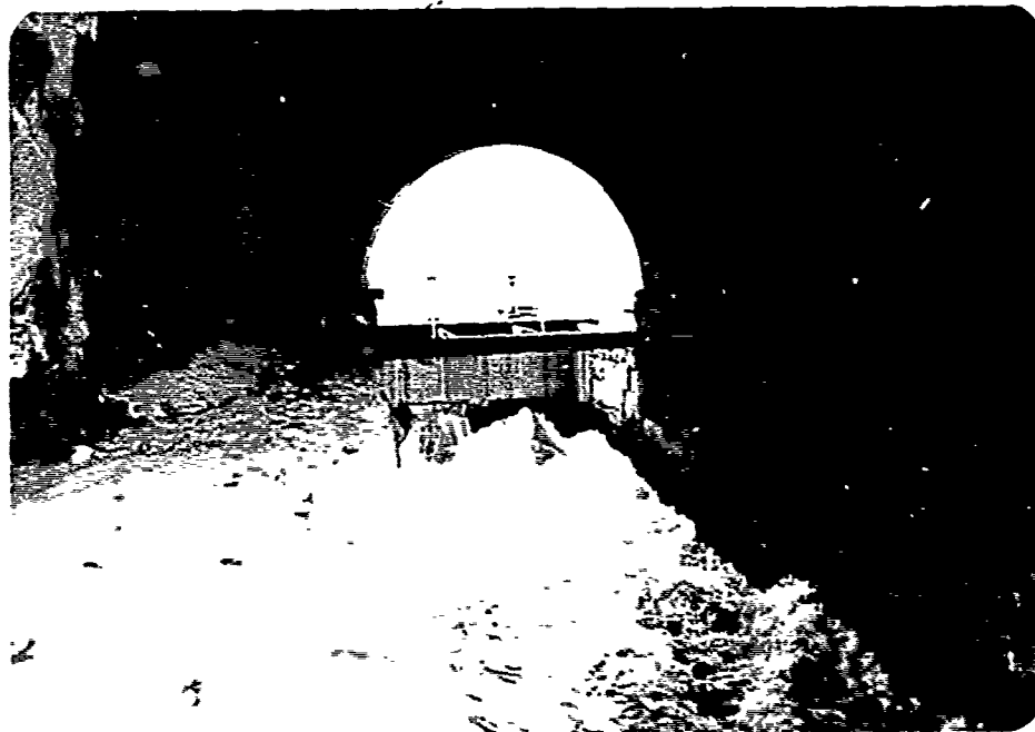
Southern Service Spillway-Looking Upstream
