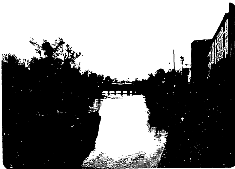
Railroad Bridge Upstream of Dam which Restricts Flow
