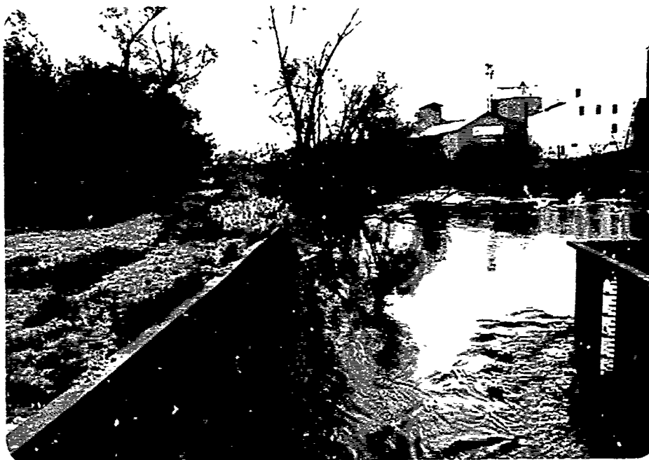
Entrance Channel Looking Upstream-Note trees Hanging Over Approach Channel
