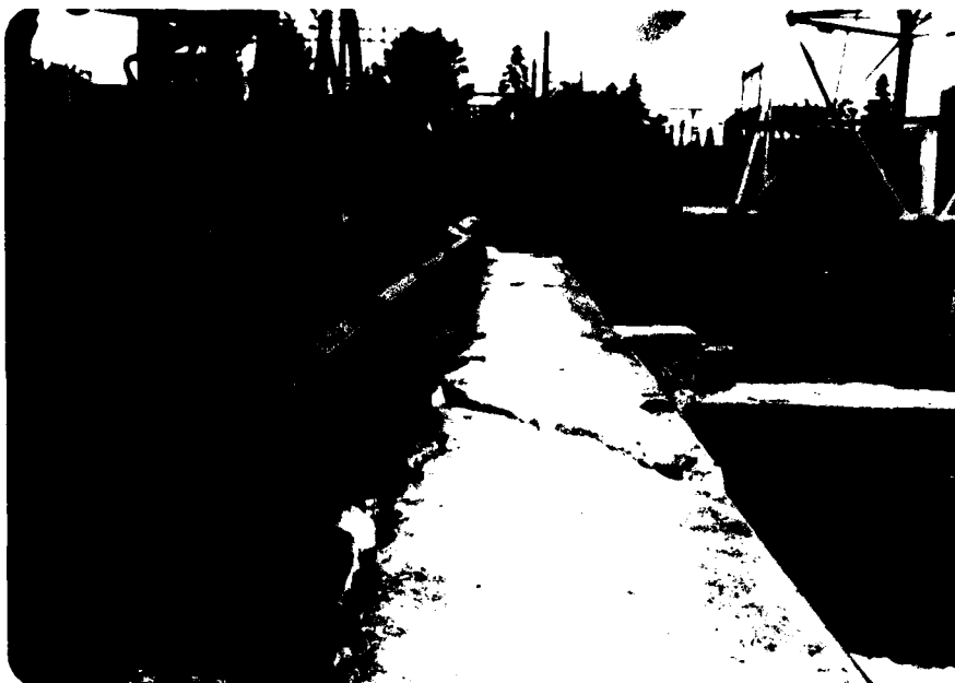
3. Cracked walkway with rail lashed to operating mechanism at sluice gate structure.
