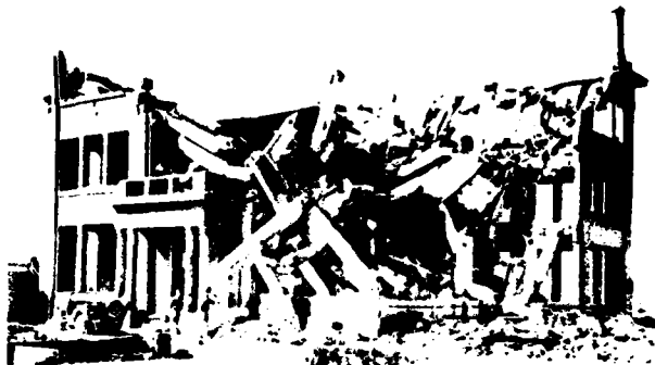
Fig. 3. Hiroshima ( \sim 14 kt, 567 m HOB) Heavy reinforced concrete 3-story building near ground zero.
