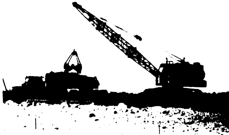
Figure 33. Backfilling the gasoline trench from the road with a clam shell.
