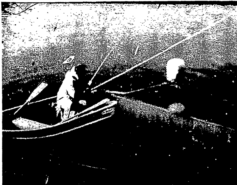
Figure 10. Window-Shade Drogue Stationary in Water
