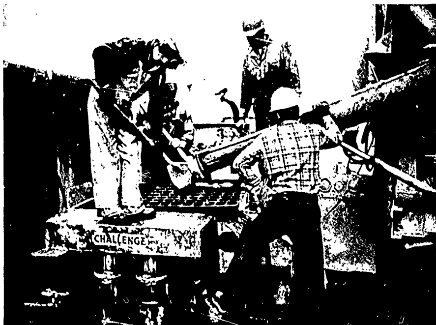
Figure 99. Fiber concrete pumping operation, Libby Dam
