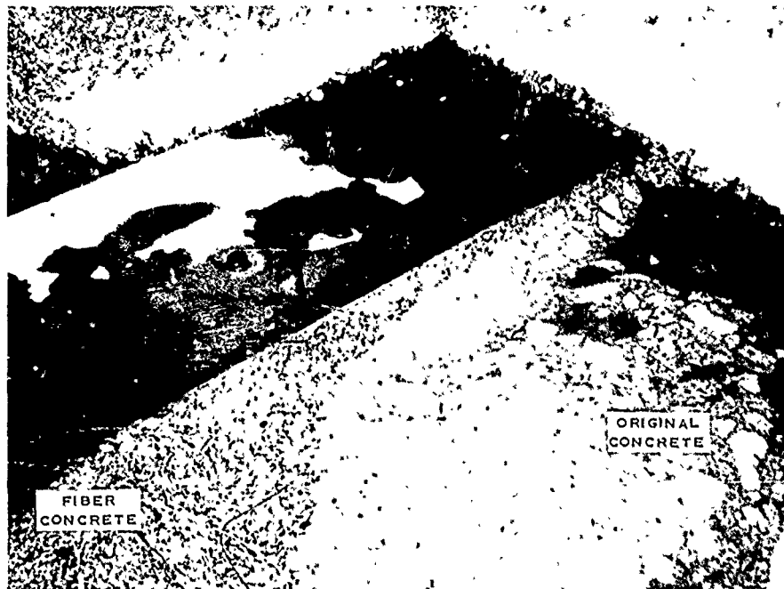
Figure 64. Erosion extending through the fiber concrete (along the steel plate) and into the original concrete, Upper St. Anthony Falls Lock
