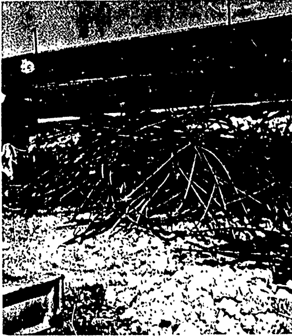
a. Loose reinforcement removed from right basin
