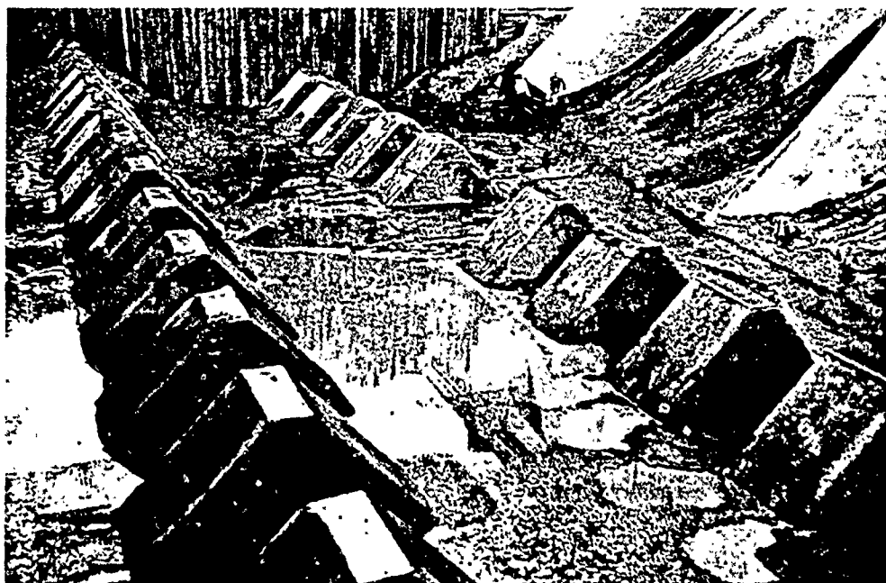
a. Baffle and deck erosion
