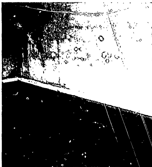
Figure 49. Different views of concrete deterioration along waterline, Lac Qui Parle Dam (from St. Paul District 1974)
