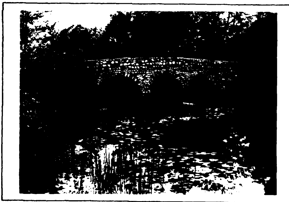
12. BRIDGE ON WELDON BROOK ABOUT 150 FEET DOWNSTREAM OF THE DAM. (5/28/80)
