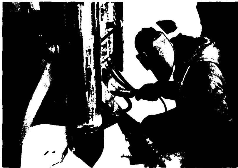
Fig. B-12. Each casing length had to have a continuous weld at each end. Note asbestos blanket around casing.
