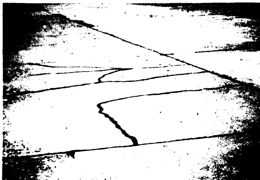
Figure B-122. Low severity intersecting cracks, case 2
