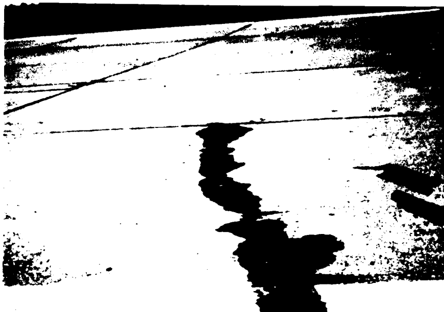
Figure B-82. Medium severity transverse crack, jointed rigid pavement, case 1
