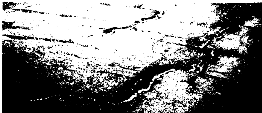
Figure B-18. High severity block cracking, case 1
