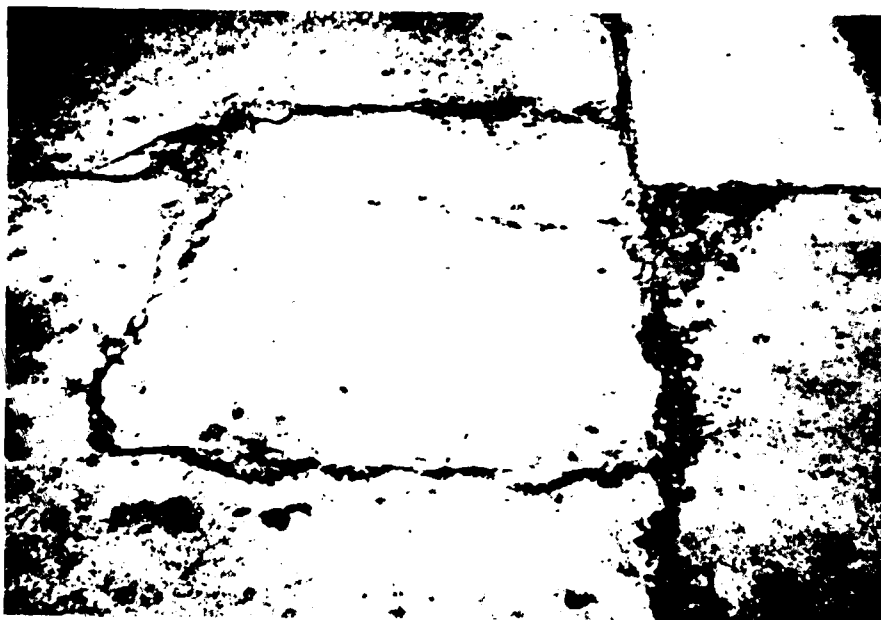
Figure B-104. High severity patch, jointed rigid pavement
