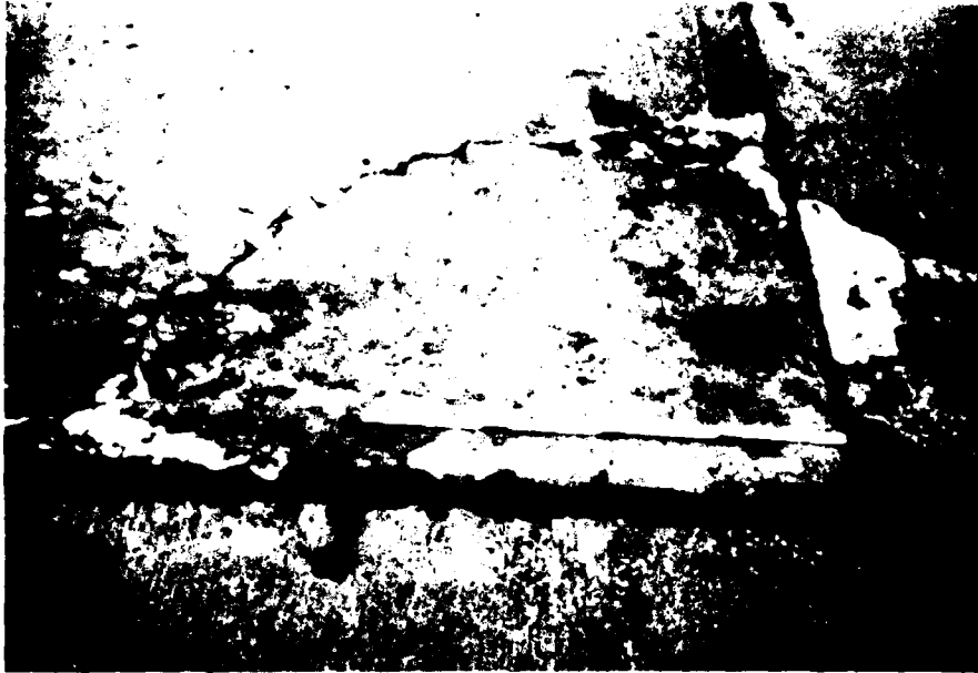
Figure B-77. High severity corner break
