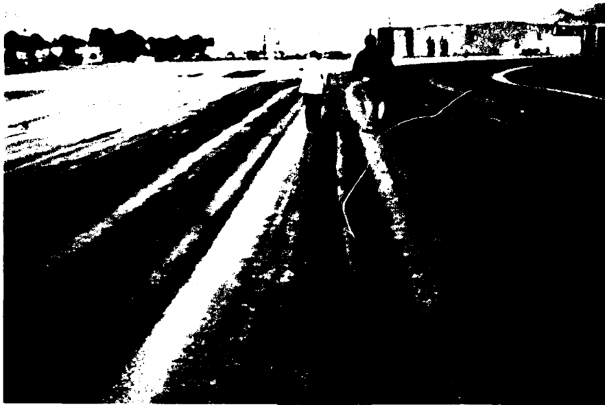
Figure B-45. Light severity patch, flexible pavement, case 1
