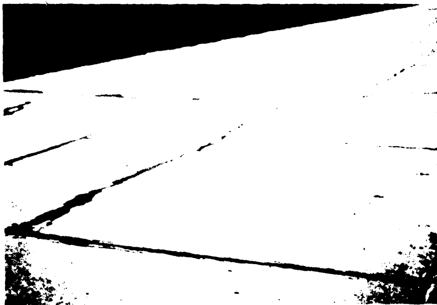
Figure B-124. Medium severity intersecting cracks, case 2
