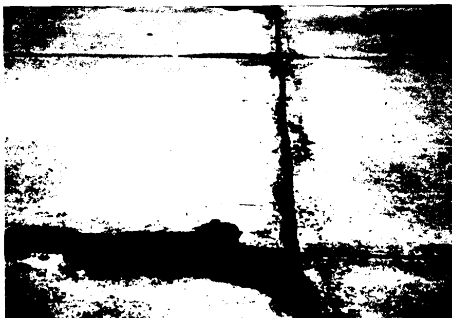
Figure B-112. Medium severity scaling
