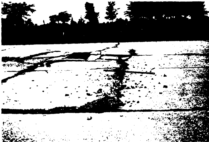
Figure B-70. Low severity blowup (Note that this would only be considered low severity if the shattering in the foreground was the only part existing and the foreign material removed.)
