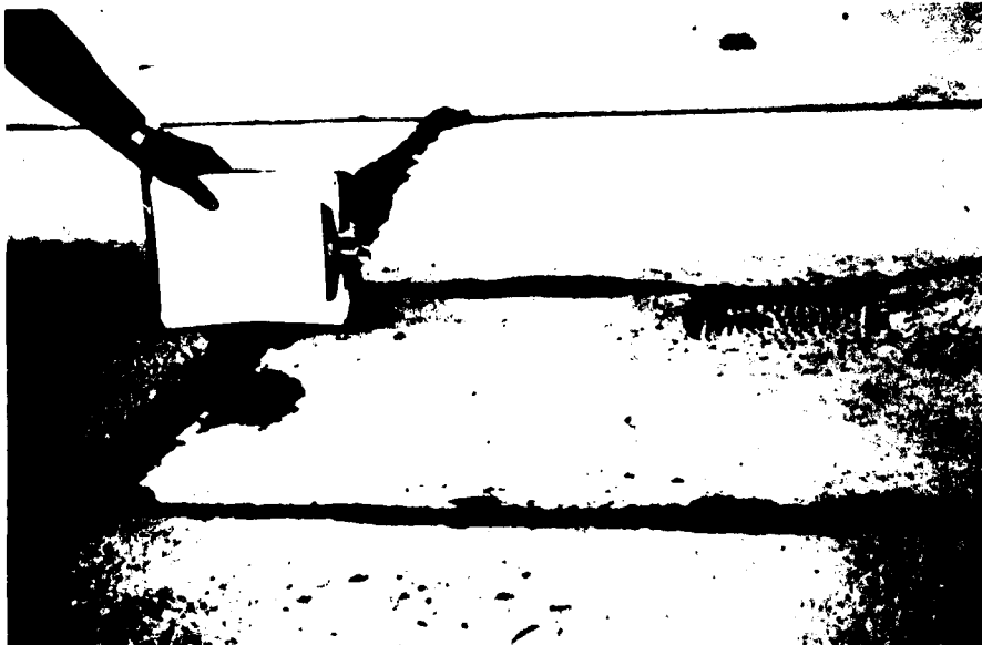
Figure B-115. Low severity settlement (3/8 in.) on apron, case 1
