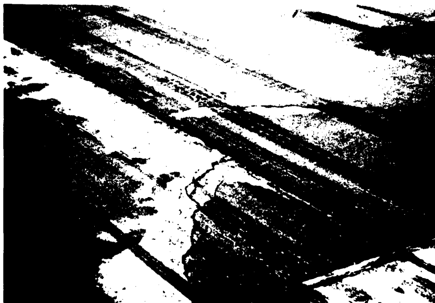
Figure B-76. Medium severity corner break, case 2
