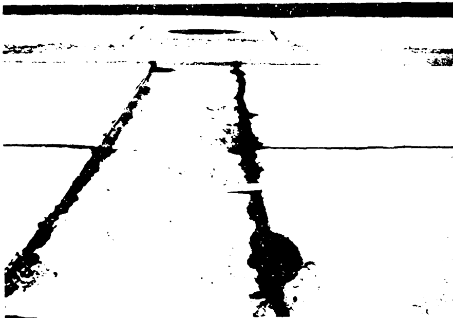
Figure B-103. Medium severity utility cut
