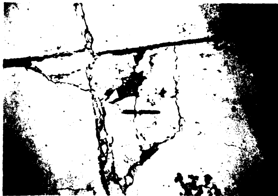
Figure B-141. High severity corner spall, case 2
