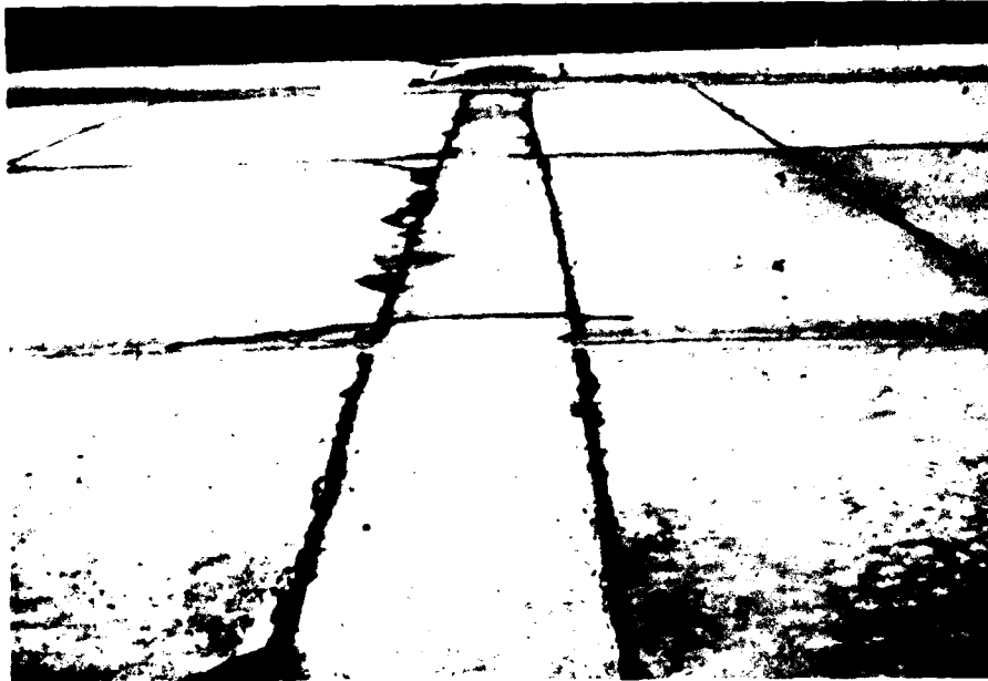
Figure B-102. Low severity utility cut
