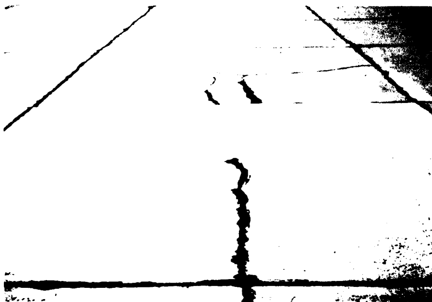
Figure B-101. Low severity patch, jointed rigid pavement, case 2
