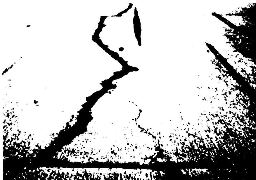
Figure B-85. High severity longitudinal crack, jointed rigid pavement, case 1
