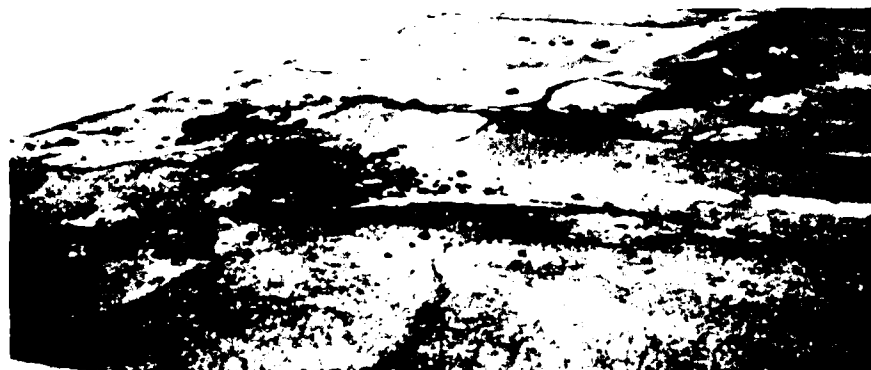
Figure B-63. High severity shoving
