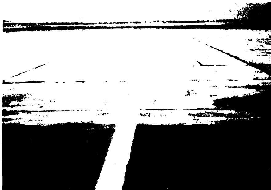
Figure B-30. Low severity joint reflection cracking
