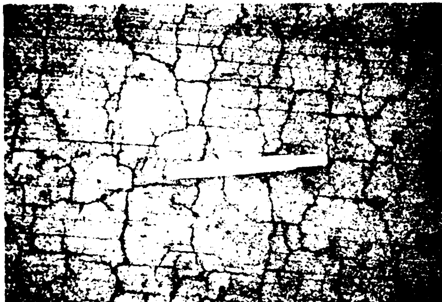
Figure B-111. Low severity crazing
