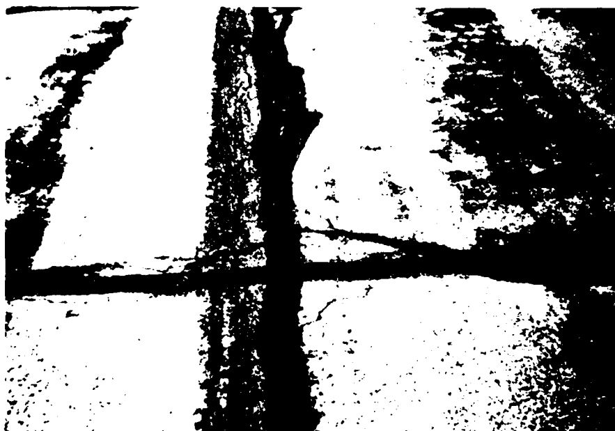
Figure B-35. Medium severity joint reflection cracking, case 3
