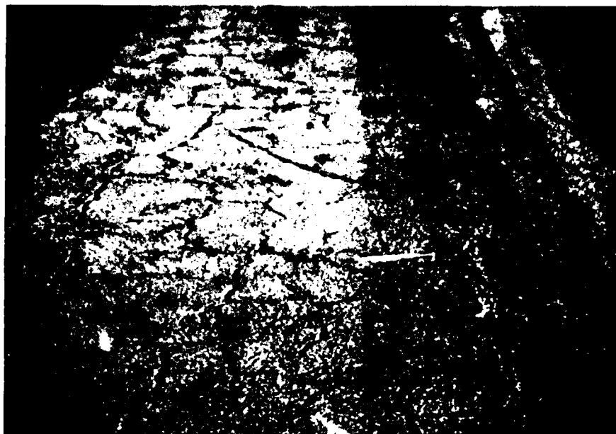
Figure B-20. High severity block cracking, case 3
