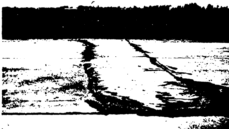
Figure B-71. Medium severity blowup
