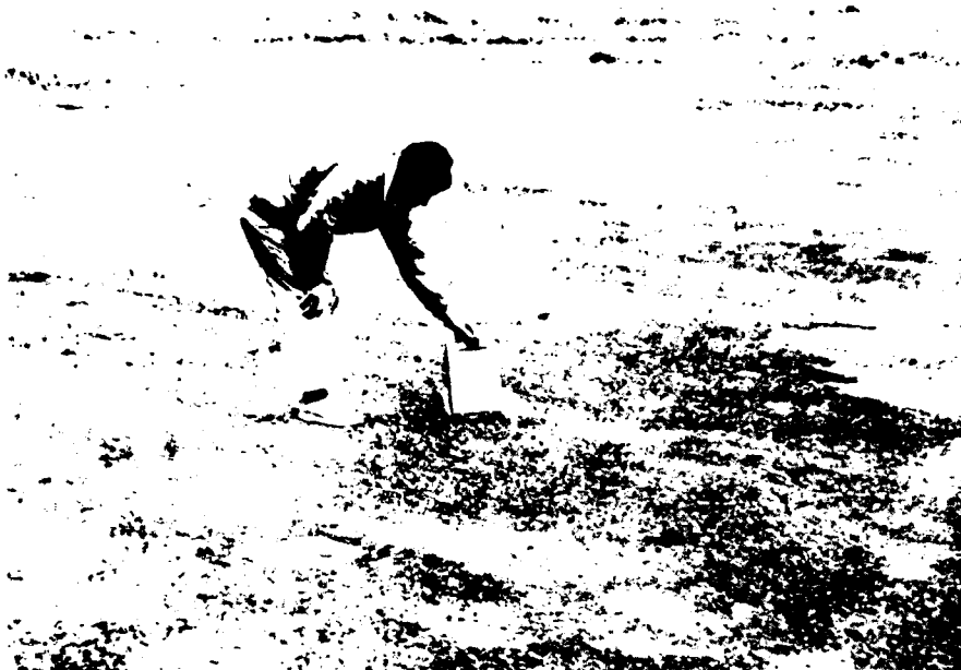
Figure B-55. High severity raveling/weathering, case 1
