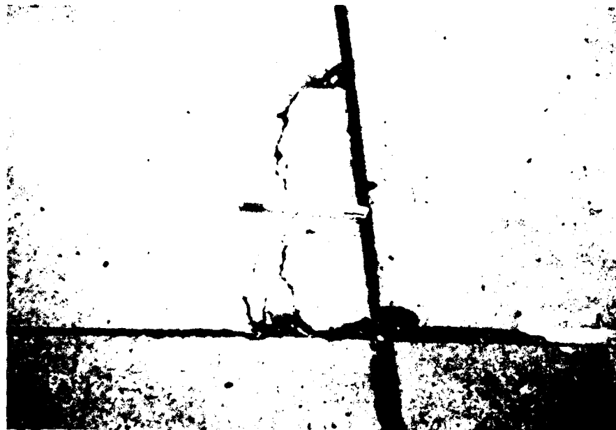
Figure B-140. High severity corner spall, case 1
