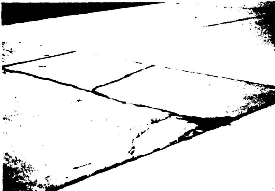
Figure B-123. Medium severity intersecting cracks, case 1
