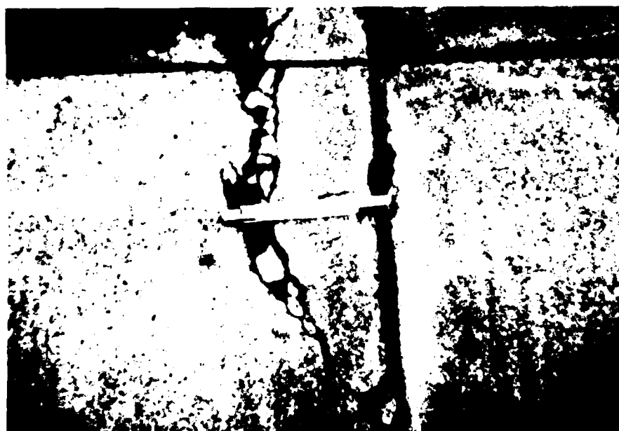
Figure B-139. Medium severity corner spall, case 2
