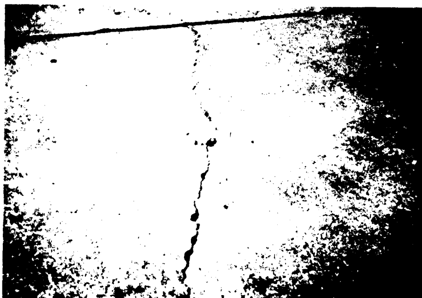
Figure B-83. Medium severity transverse crack, jointed rigid pavement, case 2
