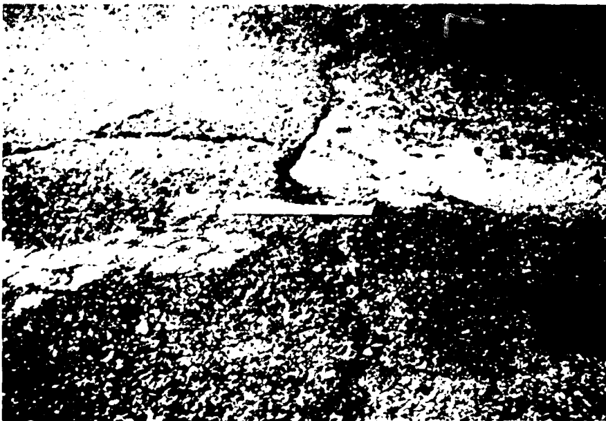
Figure B-42. High severity longitudinal crack, flexible pavement
