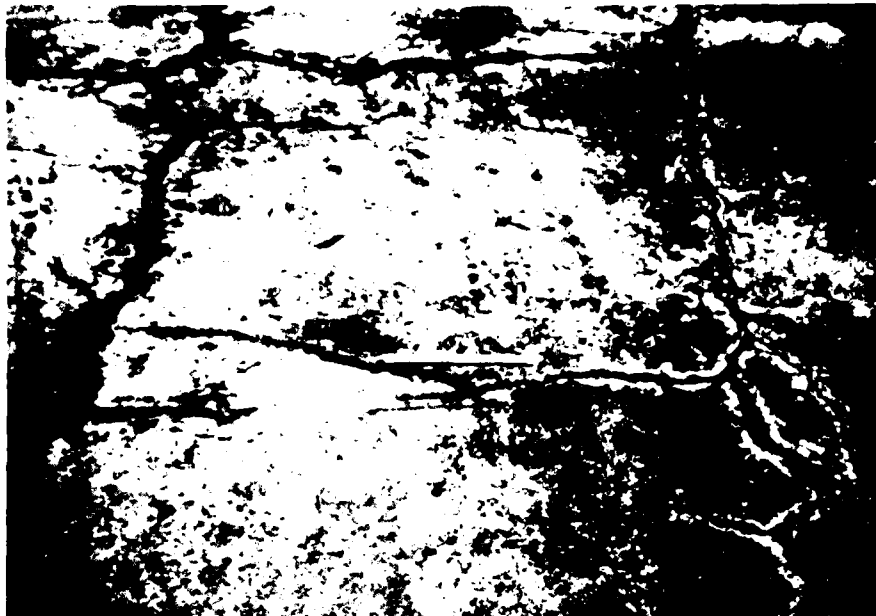
Figure B-16. Medium severity block cracking, case 1
