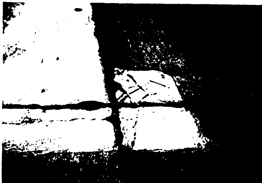
Figure B-98. Medium severity small patch, jointed rigid pavement, case 2
