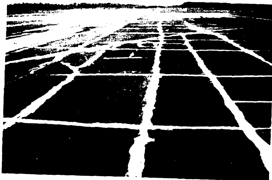
Figure B-13. Low severity block cracking, filled cracks, case 1
