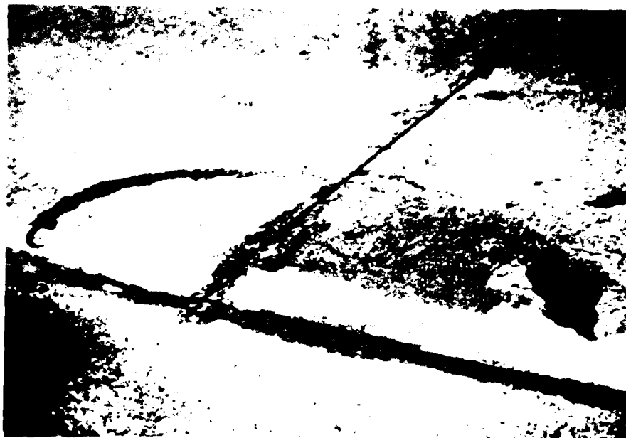
Figure B-106. Pumping (Note fine material on surface that has been pumped out causing corner break.)
