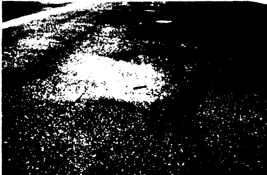
Figure B-26. Medium severity depression ( > 1/2 in.), case 2
