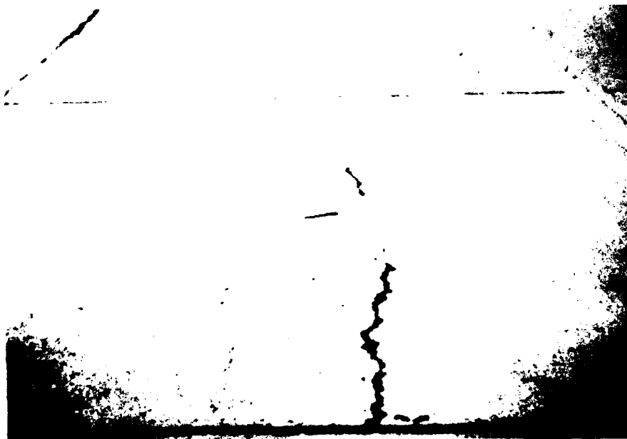
Figure B-81. Medium severity longitudinal crack, jointed rigid pavement
