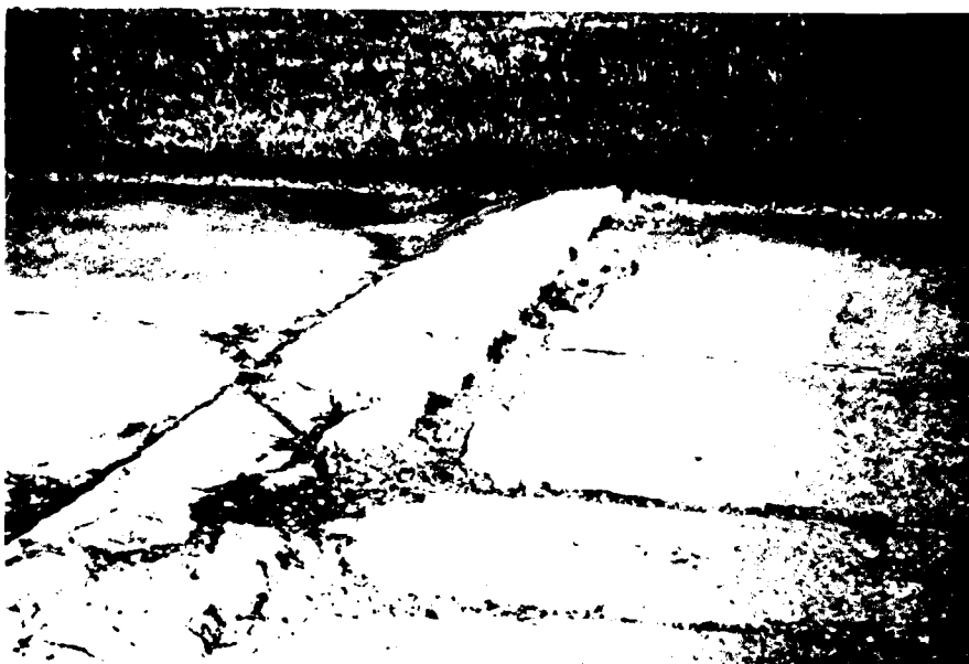
Figure B-72. High severity blowup
