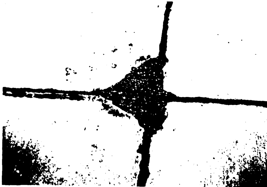
Figure B-96. Low severity small patch, jointed rigid pavement, case 2
