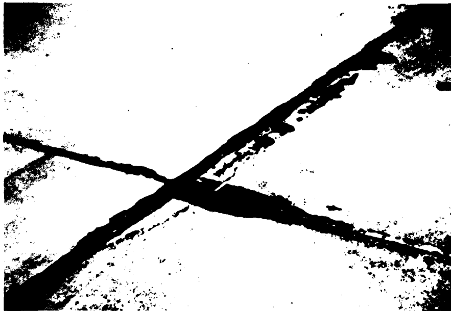
Figure B-137. Low severity corner spall, case 2
