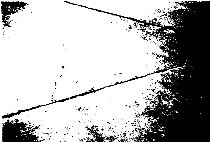
Figure B-80. Low severity diagonal crack, jointed rigid pavement
