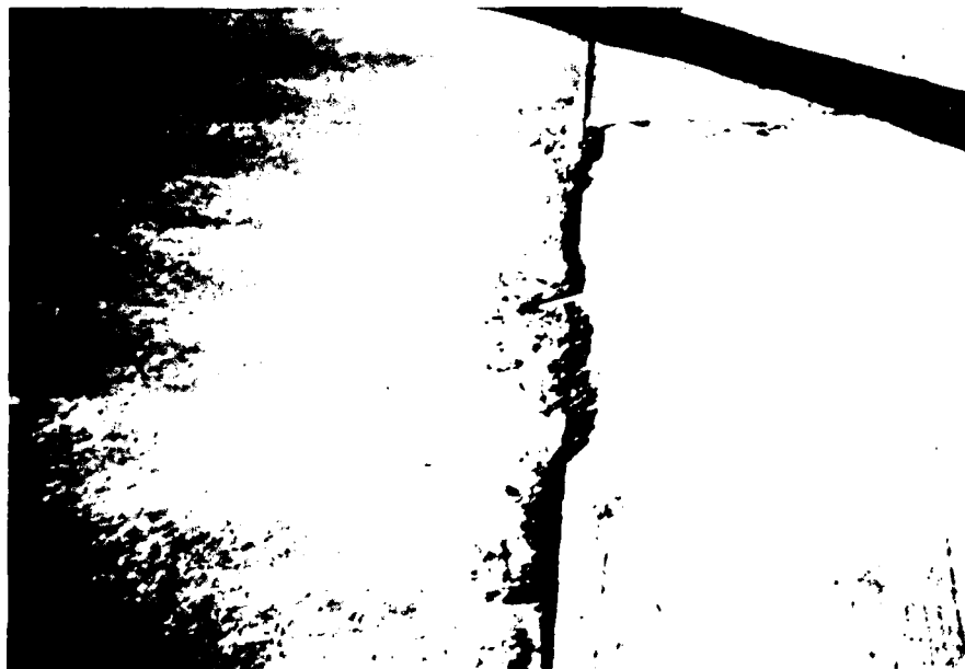
Figure B-135. High severity joint spall, case 2
