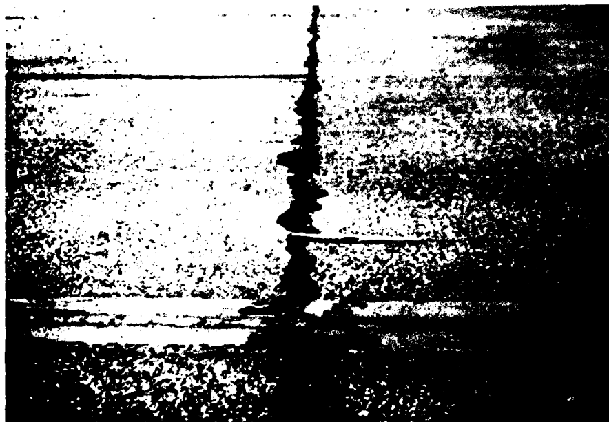
Figure B-33. Medium severity joint reflection cracking, case 1
