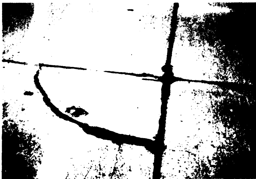
Figure B-74. Low severity corner break, case 2
