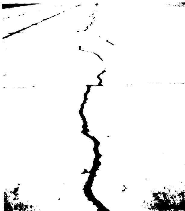
Figure B-79. Low severity filled longitudinal cracks, jointed rigid pavement
