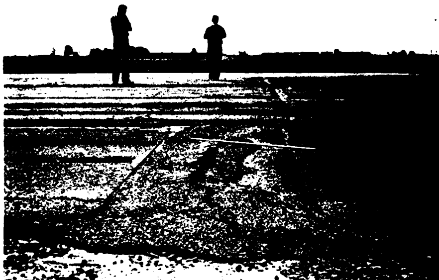
Figure B-49. High severity patch, flexible pavement
