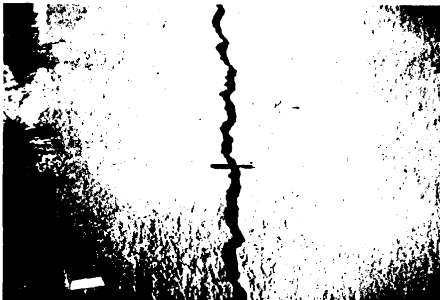
Figure B-86. High severity longitudinal crack, jointed rigid pavement, case 2
