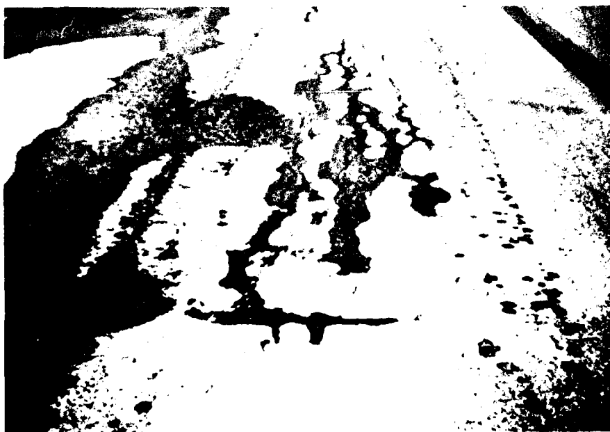
Figure B-2. Low severity alligator cracking, case 2
