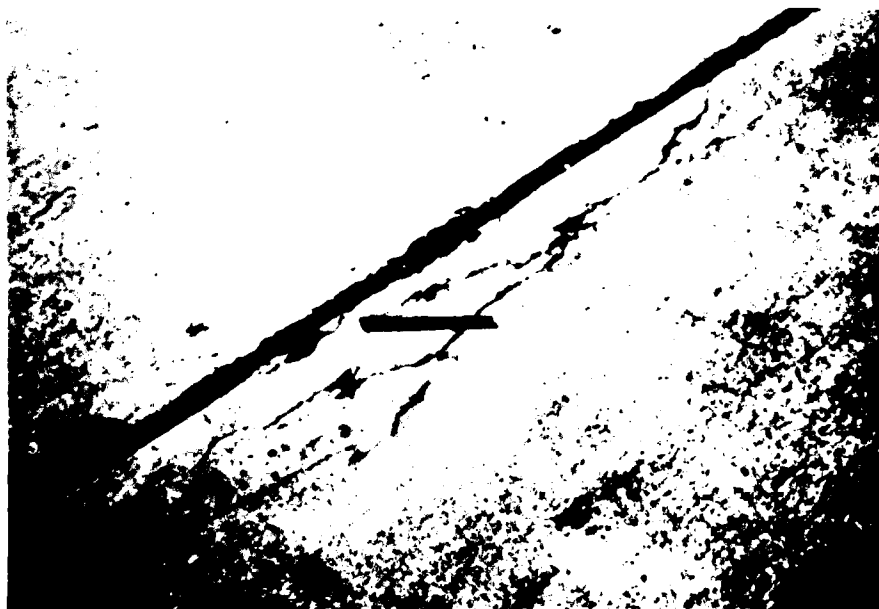
Figure B-89. Medium severity "D" cracking, case 2
