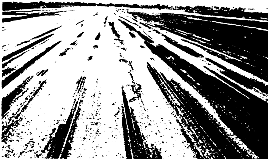
Figure B-38. Low severity longitudinal cracks, approaching medium, flexible pavement
