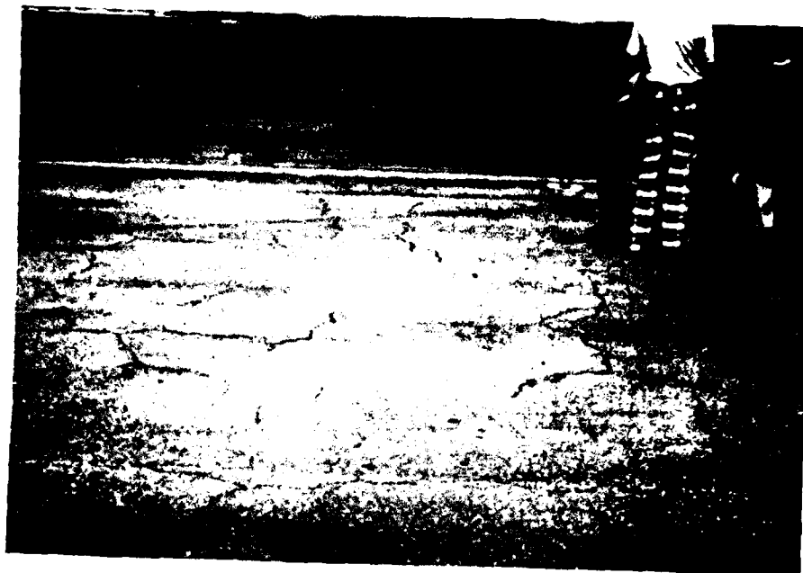
Figure B-12. Low severity block cracking
