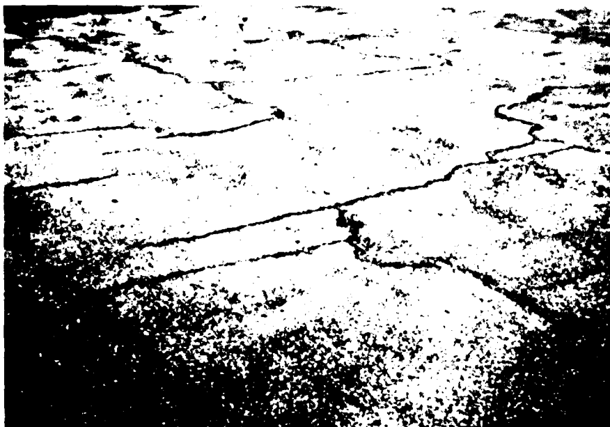
Figure B-17. Medium severity block cracking, case 2
