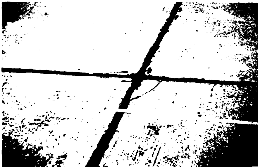
Figure B-136. Low severity corner spall, case 1
