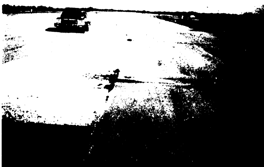
Figure B-47. Light severity patch with medium severity portion, flexible pavement
