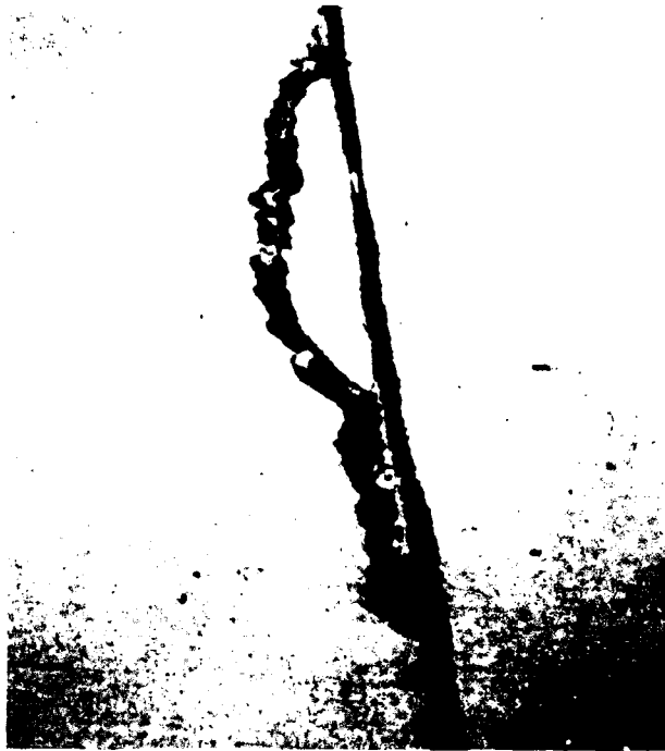
Figure B-131. Low severity joint spall, case 3
