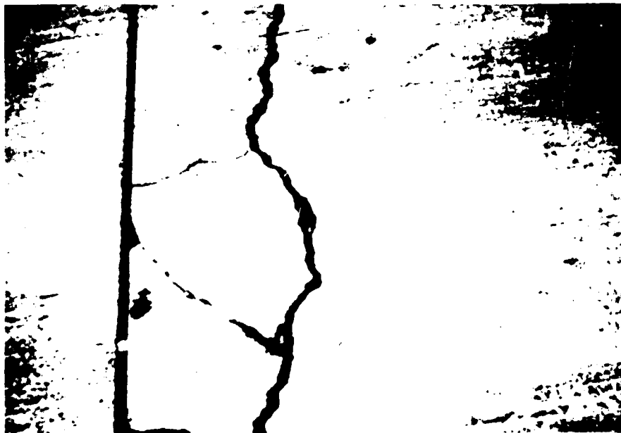
Figure B-133. Medium severity joint spall, case 2
