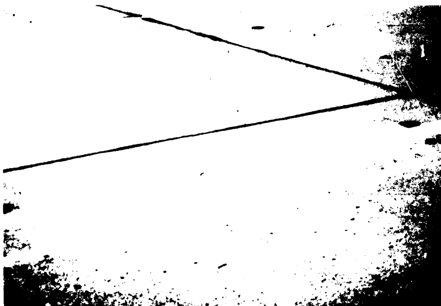
Figure B-127. Shrinkage crack, case 2
