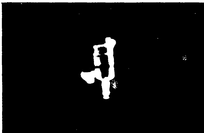
Figure 6. Good steam trap in IR viewer. Outlet line is cooler than inlet.
