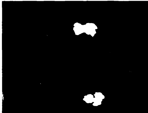
Figure 4. IR view of over-heated fuse holders in sub-station. New equipment made possible these views on a sunlit day.
