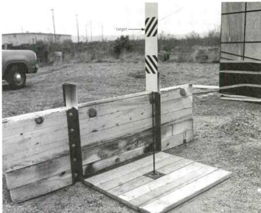
Figure 13. Timber headwall and roof without soil berm.
