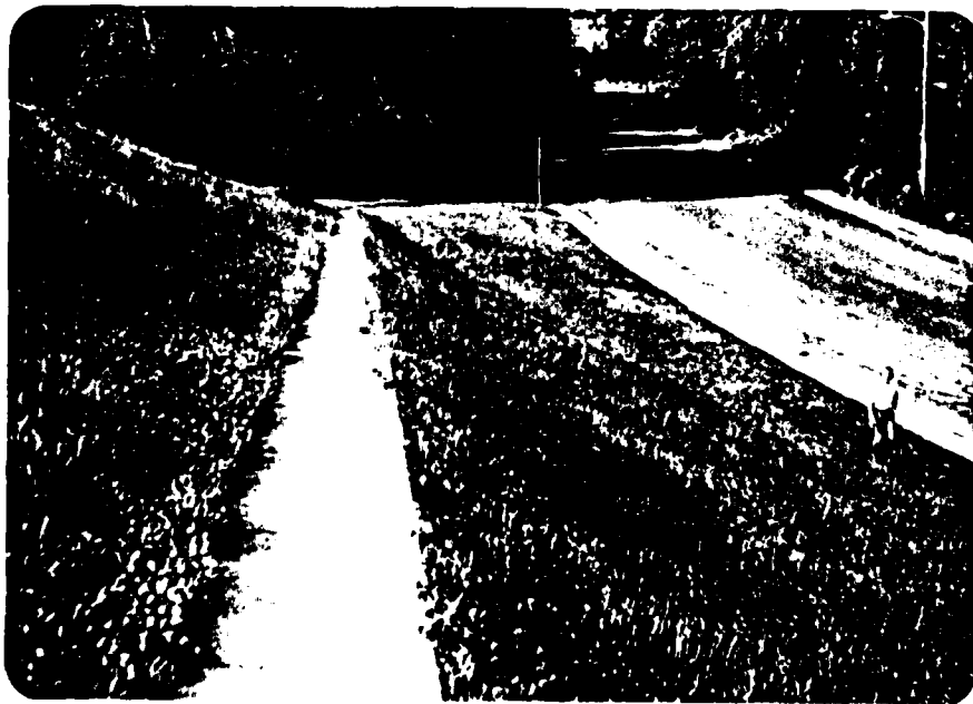
F. Southwest Corner of Embankment- Saturated Soil at Toe where man stands.
