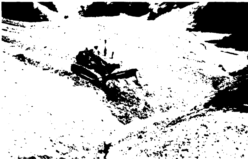
Figure 9. A bulldozer striking off the mine spoil ridges prior to revegetation
