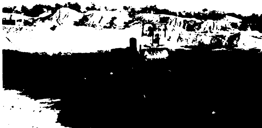
Figure 26. Spreading dredged material on plots
