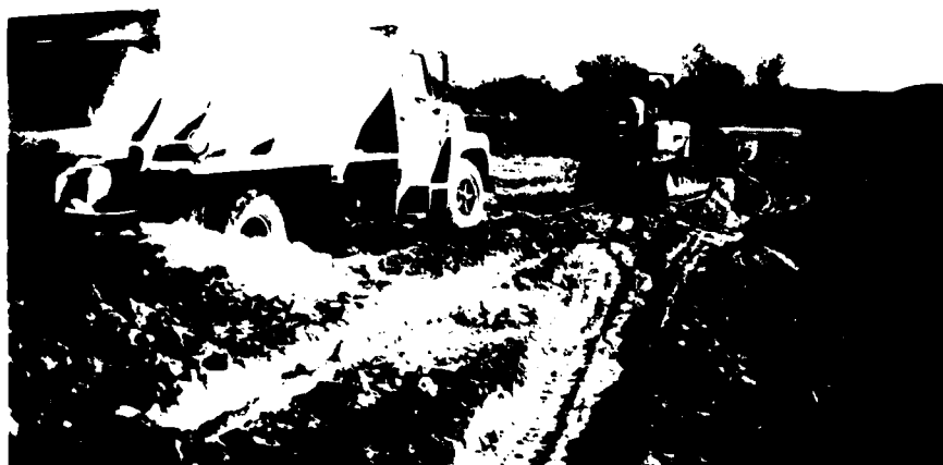
Figure 25. Spreading agricultural ground limestone on the dredged material in plot III
