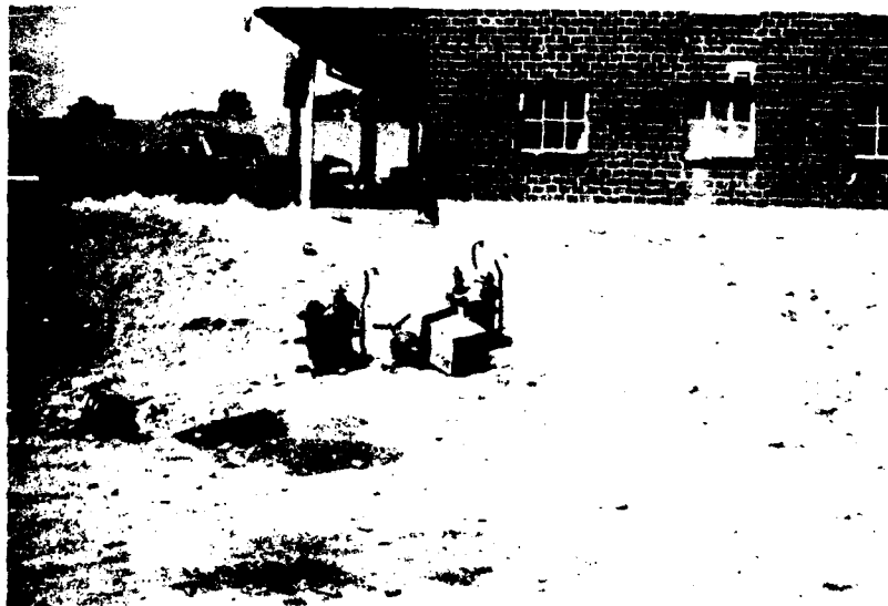
Figure 8. Electrical shop transformers -- Installation B.
