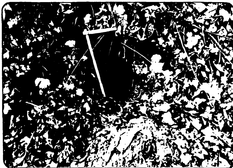
PHOTO 7. Close-up View of Rodent Hole at Toe of Slope, Approximate Station 1 + 00
