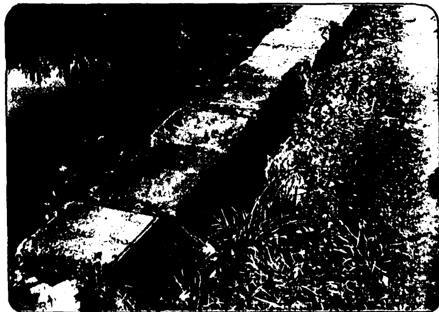
PHOTO 6. Close-up View of Slope Protection on Upstream Face (at the normal pool level)
