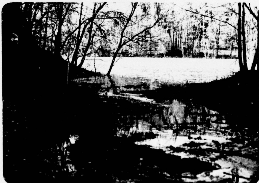
Photograph No. 2 Emergency spillway approach channel.
