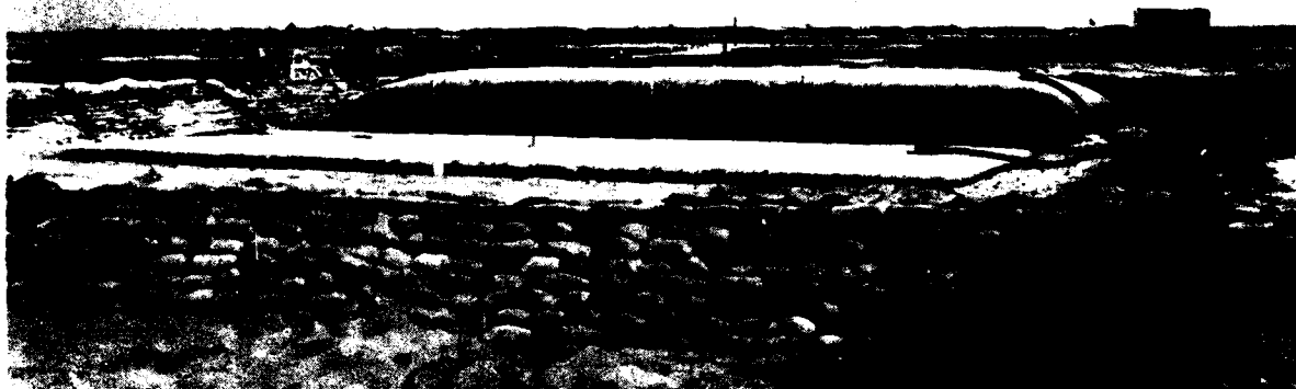
Dikes constructed to protect petroleum supplies at Tuy Hoa Air Base
