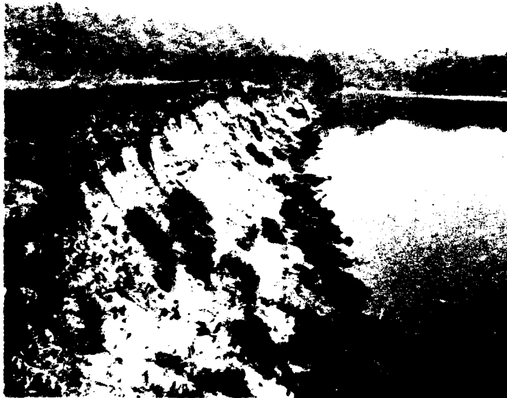
Figure 65. Sloughing on a partially vegetated or barren bank.
