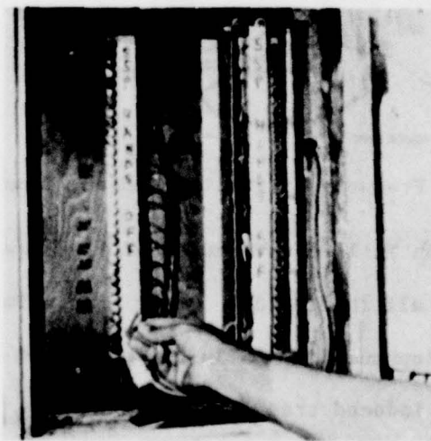
Figure 3B. Interior View of the Terminal Showing Carbon Block Holders (Vertical Strip, Right Side)
