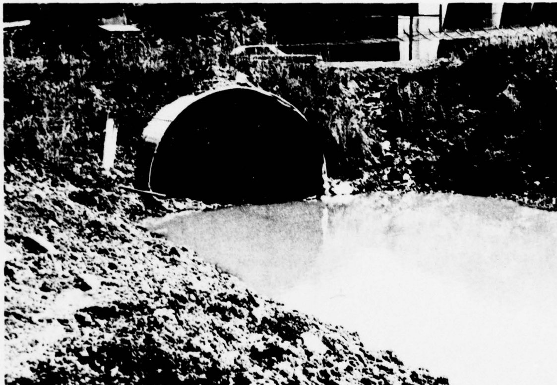
VIEW OF STILLING BASIN AND CMP WHICH DISCHARGES UNDER ROADWAY
