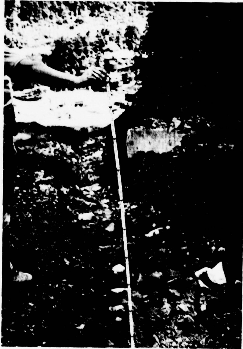
EROSION ON FACE OF DAM LOCATED JUST LEFT OF CONCRETE SPILLWAY
