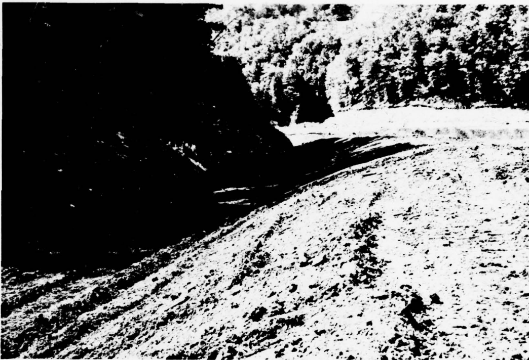
NEW DIVERSION CHANNEL BEING CUT INTO THE RIGHT ABUTMENT (LOCATION IS BETWEEN CONCRETE SPILLWAY AND RIGHT ABUTMENT)
