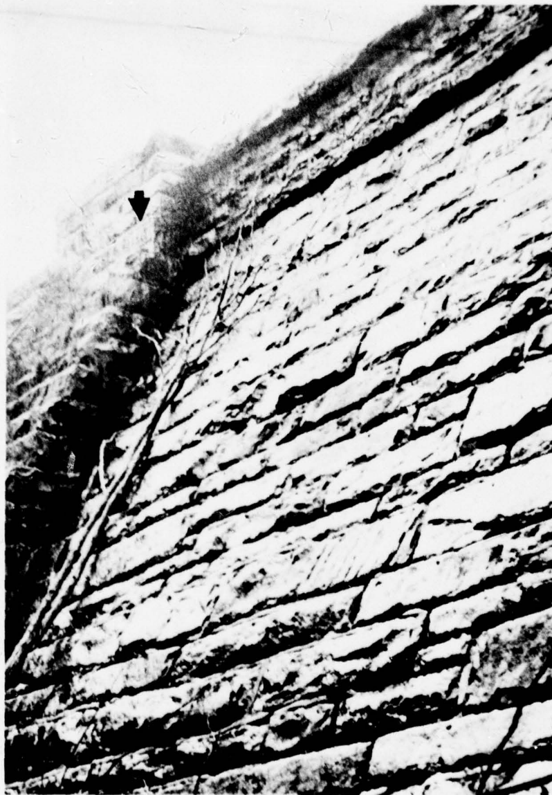
VIEW SHOWING GOOD CONDITION OF RUBBLE FACE (NOTE DATE BLOCK - ARROW)
