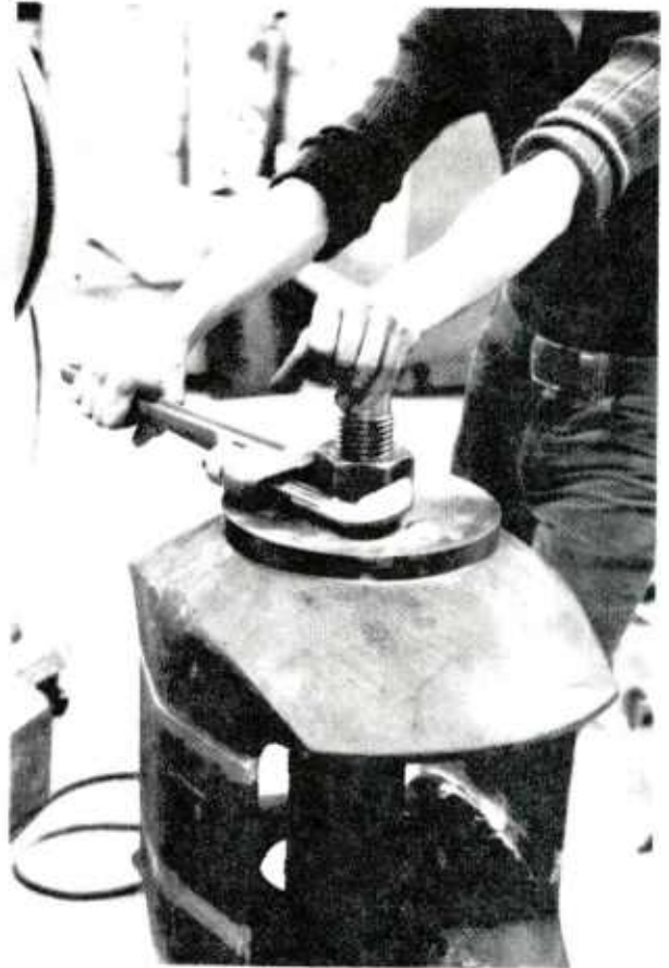
Figure 13. Muzzle brake assy - lock
