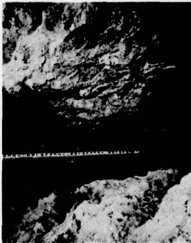
a. Rainfall erosion tunnel sta 138+00 (middle slope), 26 March 1960
