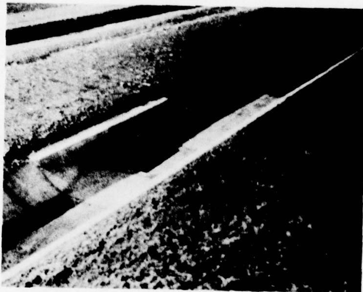
b. Completed berm ditch paving
