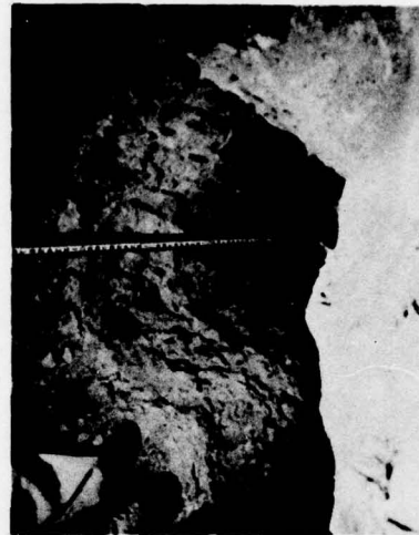
d. Rainfall erosion tunnel sta 144+00 (lower slope), 26 March 1956
