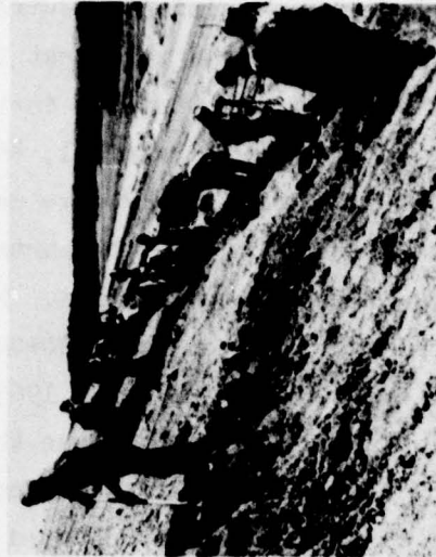
d. Compacting backfill with pneumatic tampers, 13 May 1960
