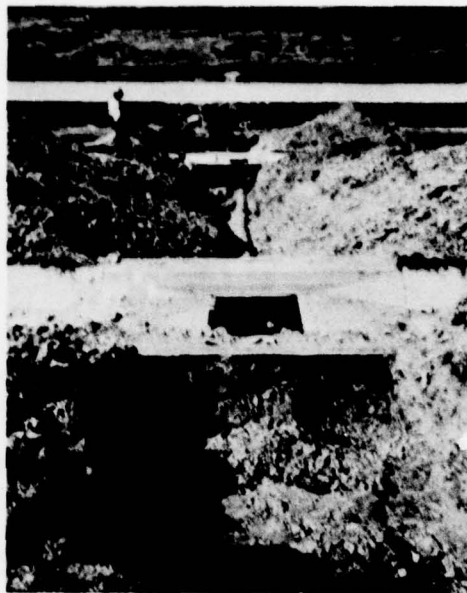
b. View downstream of excavation around concrete slope drain pipe and drop inlet, 26 March 1960
