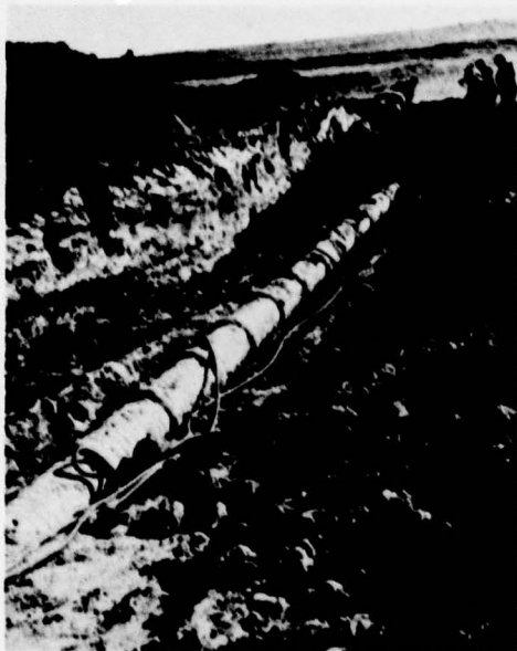
c. Backfilling around concrete slope drain pipe sta 106+00, 19 March 1960
