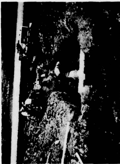
a. Excavation around concrete slope drain pipe and drop inlet
