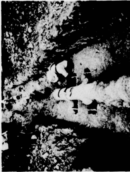
d. Repairing collar on slope drain pipe Figure 20. Repairing rainfall erosion tunnels at sta 118+00, 9 June 1958 (from File 1514-02 Subsurface Erosion, Vicksburg District)
