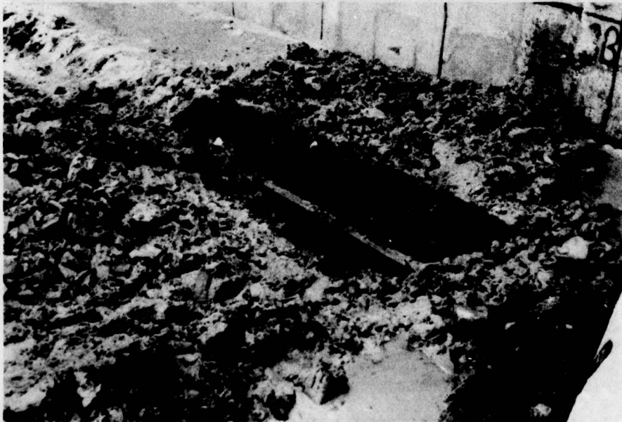
Photo 8. Portion of pile exposed by excavation
