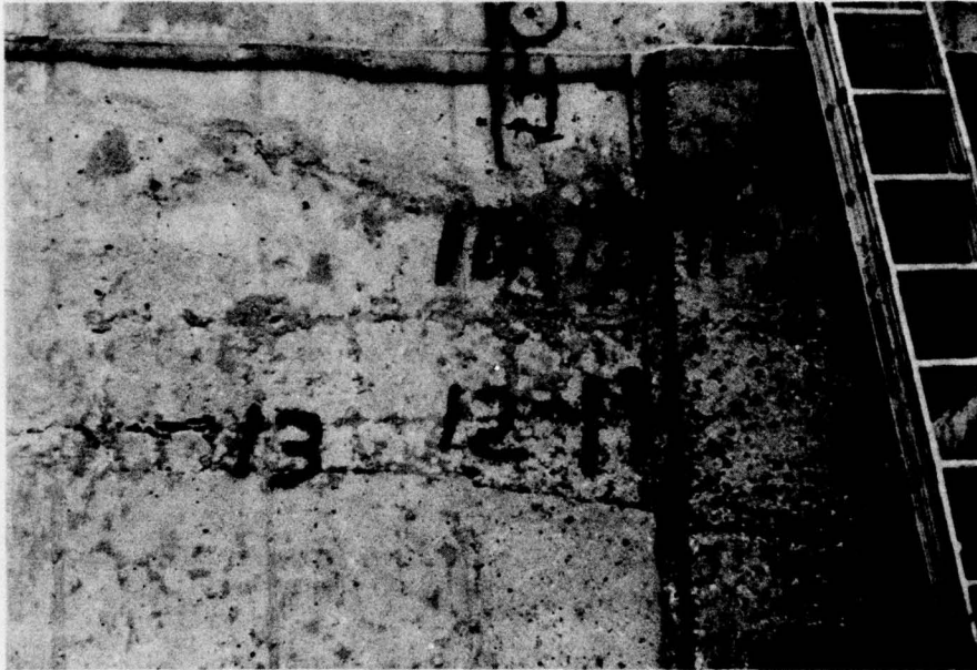
Photo 7. View showing the vertical section of concrete that houses the casing collar
