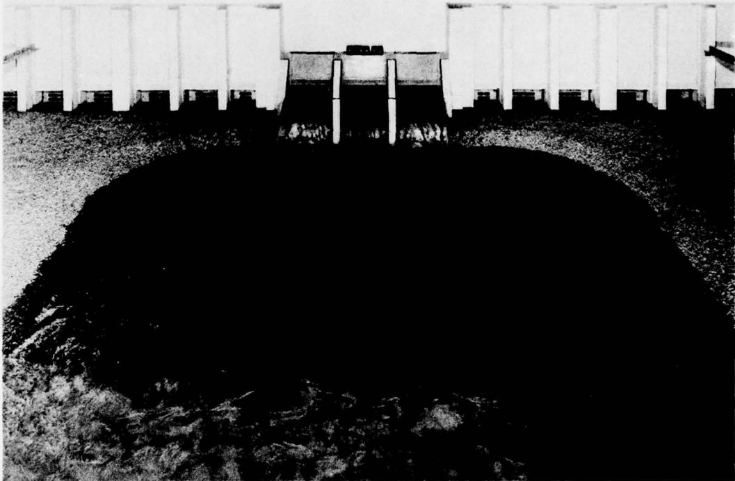
c. Discharge 12,500 cfs, tailwater el 92.8
