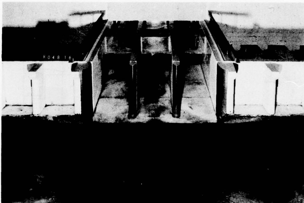
Figure 6. Type 4 approach with type 2 abutment
