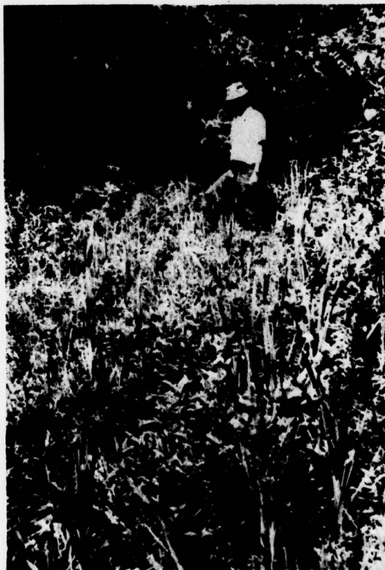
10. Overbank area below toe of dam on south side. Growth indicative of wetness.
