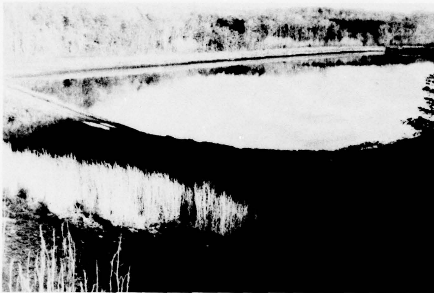
PHOTOGRAPH NO. 3 Lagoon Below Dam
