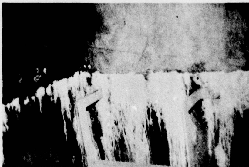
PHOTO SHOWING BLEEDING IN SECOND LEVEL OUTLET CHAMBER Photo #4
