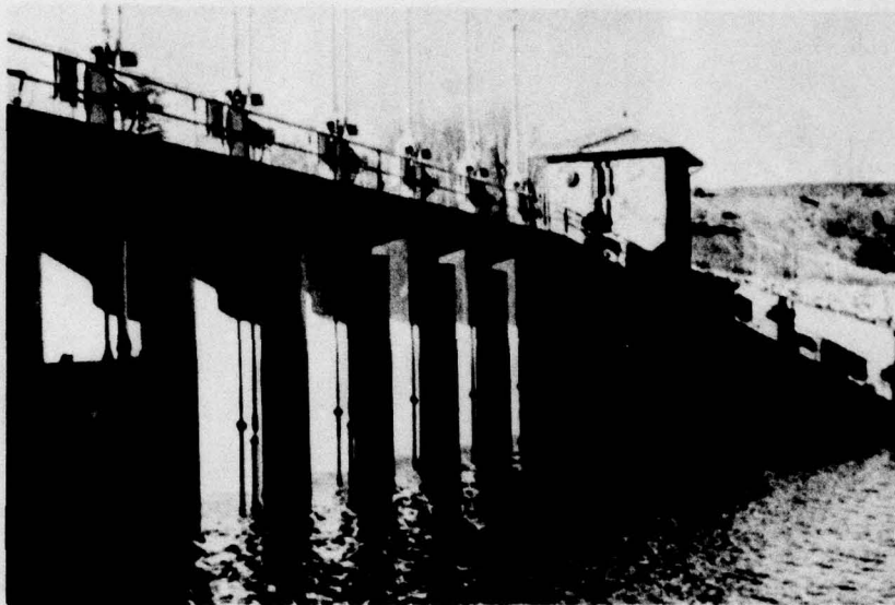
UPSTREAM VIEW OF GATES (Control Building in Background) Photo #3
