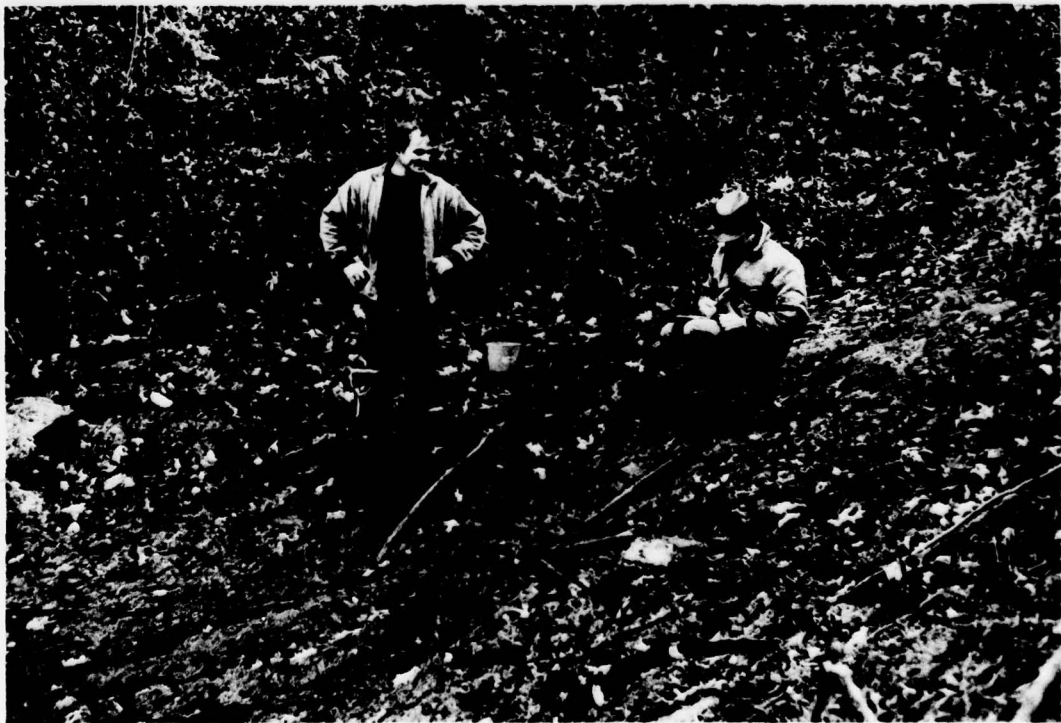
PHOTO 4. Clear Seepage Area at Downstream Right Abutment
