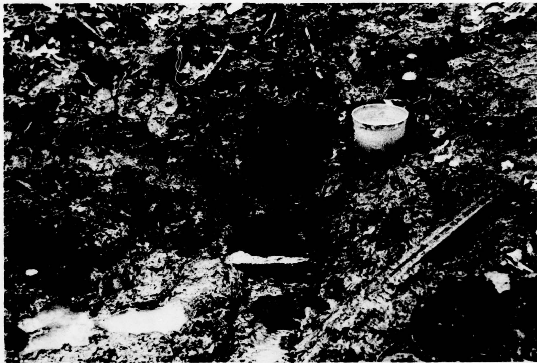
PHOTO 5. Excavated Trench in Clear Seepage Area at Right Abutment (Used to Determine Flow)
