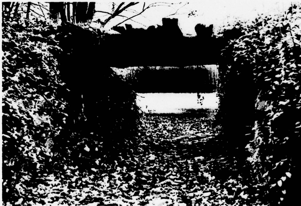
PHOTO 2. Looking Upstream at Spillway in Right Abutment of Dam
