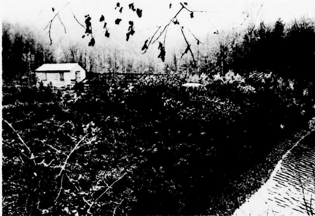
Photo 1. Outlet Works Downstream Embankment and Edge of Downstream Reservoir
