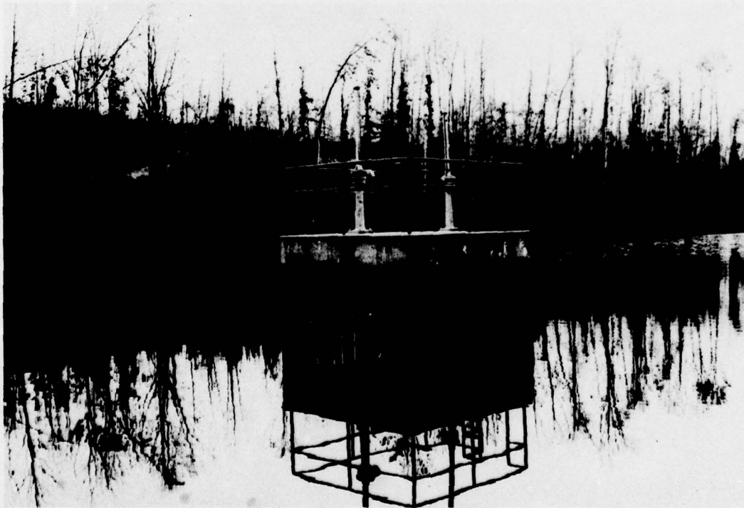
PHOTO 2. Riser of Outlet Structure in Reservoir
