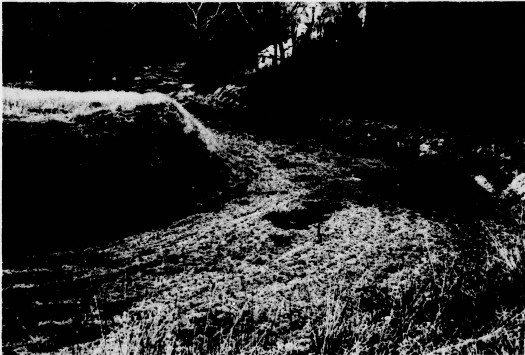
PHOTO 6. Downstream View of Emergency Spillway
