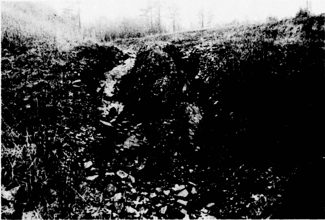
PHOTO 5. Erosion at Approach Channel to Emergency Spillway
