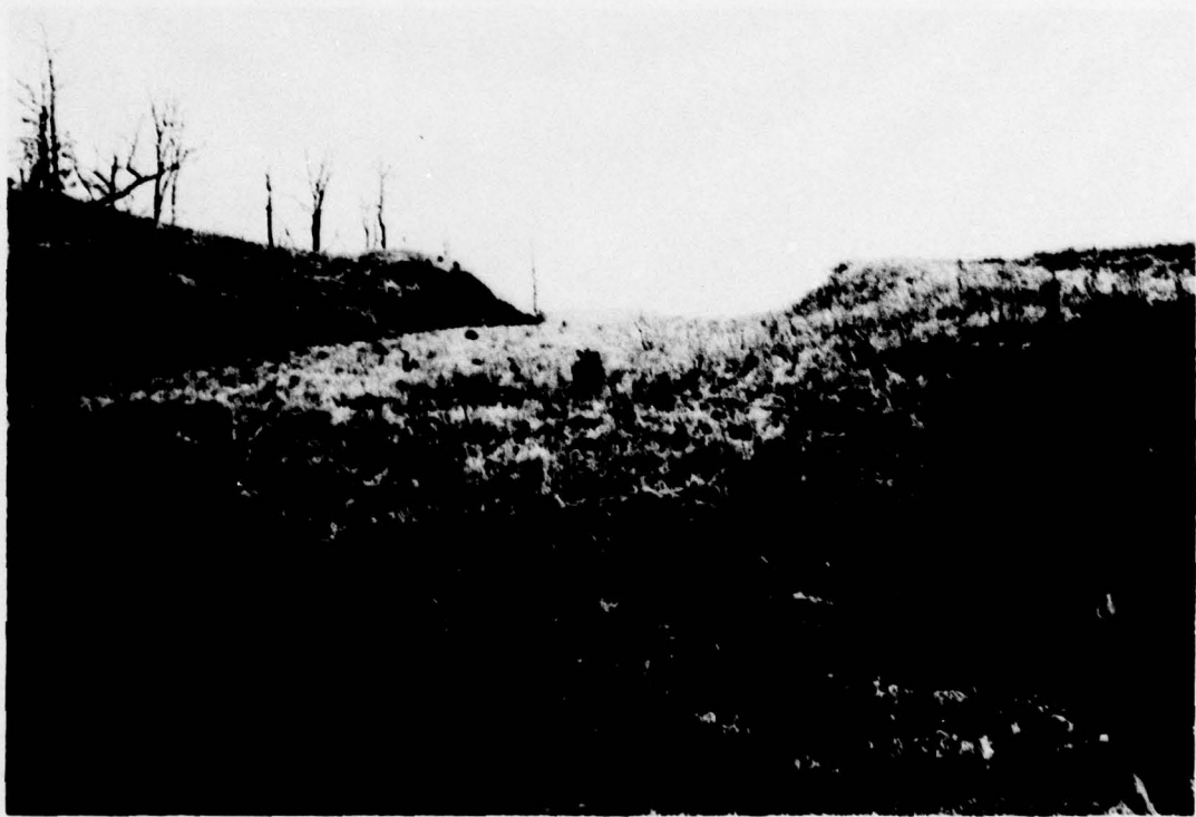
PHOTO 4. Outlet Channel for Emergency Spillway
