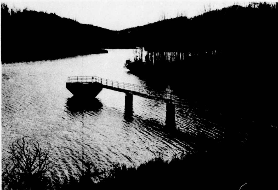
PHOTO 1. Reservoir Area, Riser and Walkway
