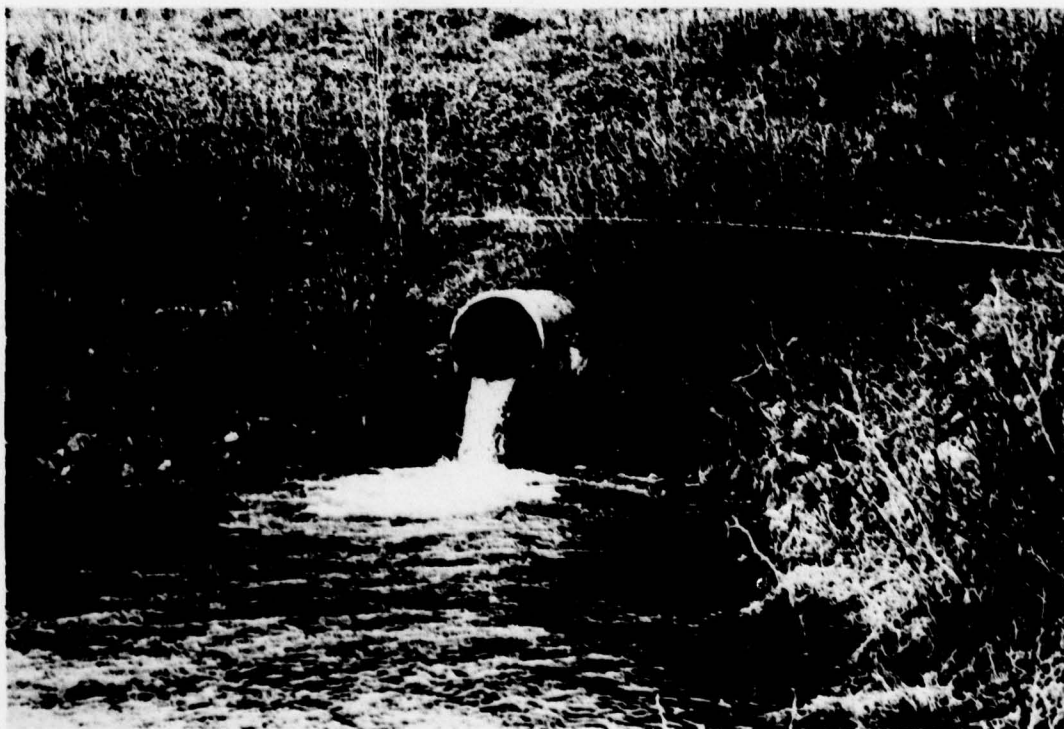
PHOTO 2. Concrete Outlet Pipe and Stilling Basin
