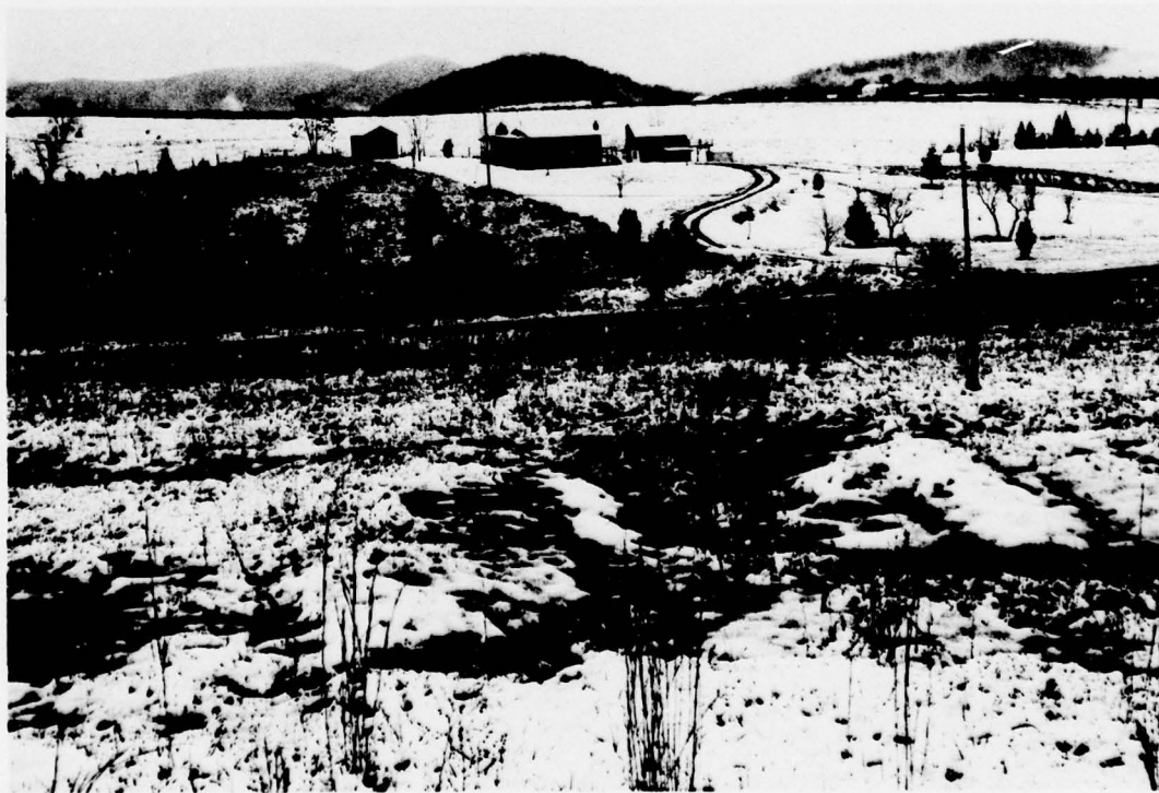
PHOTO 6. Exit Slope From Emergency Spillway
