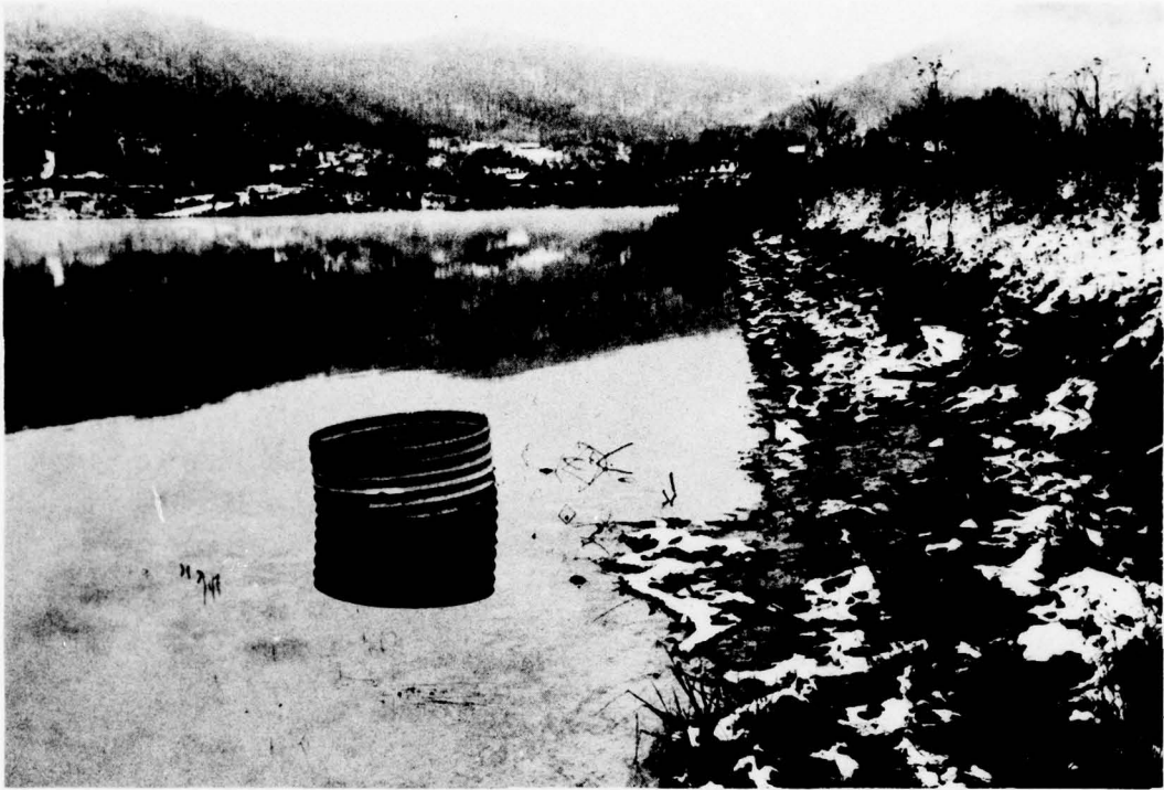
PHOTO 1. Corrugated Outlet Pipe Near Right Abutment
