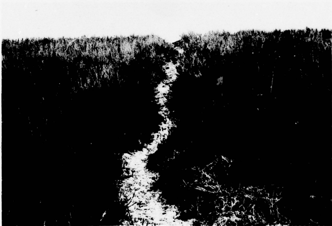
PHOTO 2. Footpath on Upstream Slope (Near Riser)
