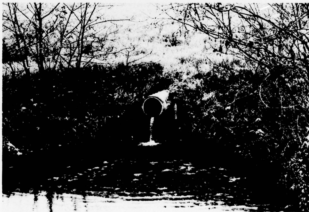
PHOTO 4. Outlet Pipe and Stilling Basin
