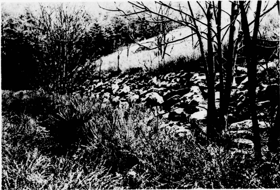
PHOTO 5. Rock Toe on Downstream Side of Dam
