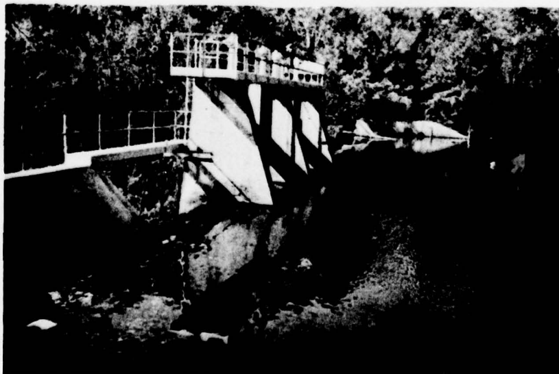
UPSTREAM VIEW OF LIFT ASSEMBLY
