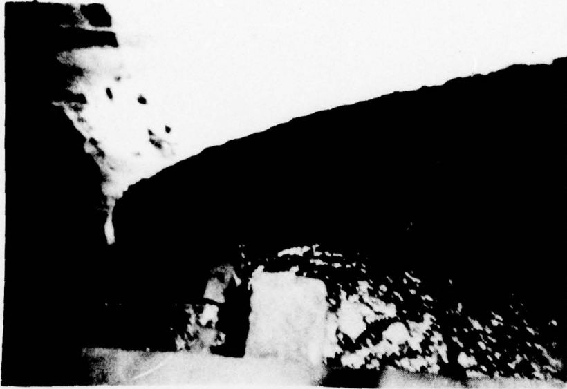
21. Seepage from wall in valve pit behind dam. Seepage discharges into stilling basin in picture No. 20 through small pipe.
