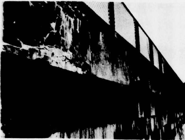
14. Detail of spalling of concrete facing on south side of downstream face of dam.
