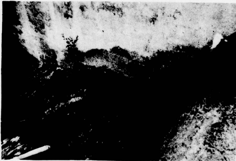
18. Detail of seepage under spillway concrete through the weathered rock joint. Seepage noted at a number of locations in spillway weir.
