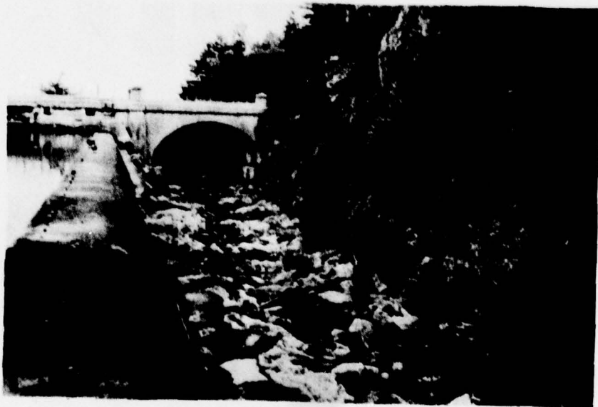
16. View down spillway side channel.
