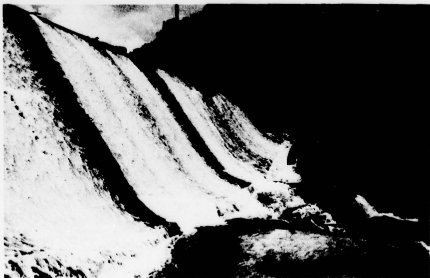
FIGURE 23 DOWNSTREAM FACE SHOWING POSSIBLE MONOLITH OFFSETS AND LEAKAGE BENEATH AND THROUGH SIDE CHANNEL SPILLWAY
