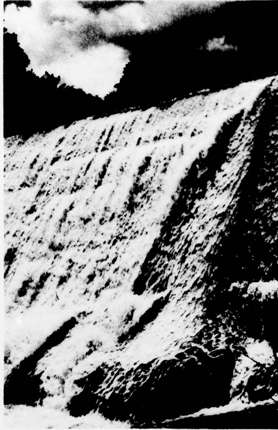
FIGURE 18 EXIT PORTALS OF TWO SLUICE PIPES ON DOWNSTREAM FACE
