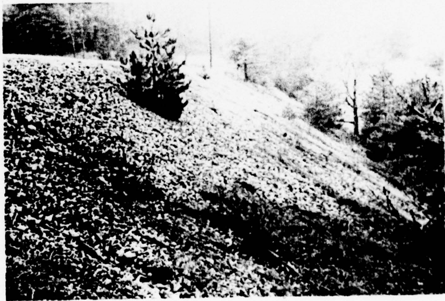
DOWNSTREAM FACE-VIEWED FROM RIGHT ABUTMENT
