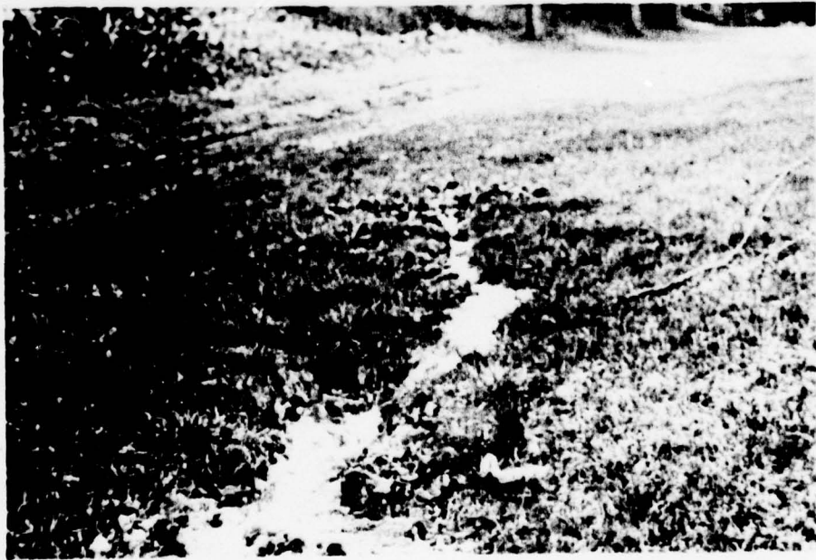
SEEPAGE, LEFT SIDE BEYOND TOE
