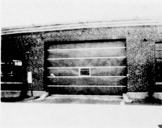
Figure 106. Insulated fiberglass overhead door at New Hampshire Highway Garage.
