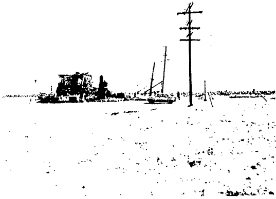
Fig. 3.9—Failure of the distribution circuit at the rear of the 4700-ft property line.
