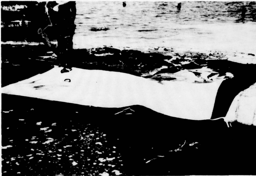
a. Cloth bags are placed empty on filter cloth
