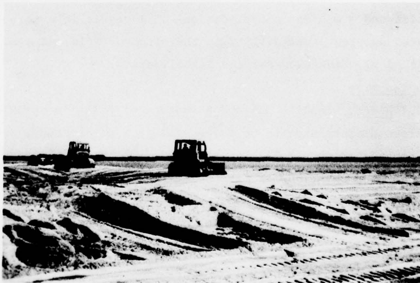
Figure 27. Site grading at the Buttermilk Sound site. Sandy substrates can often be easily manipulated to control elevation, drainage, and species diversity
