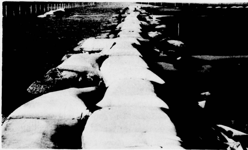
d. Dike after exposure to the elements for 2 years
