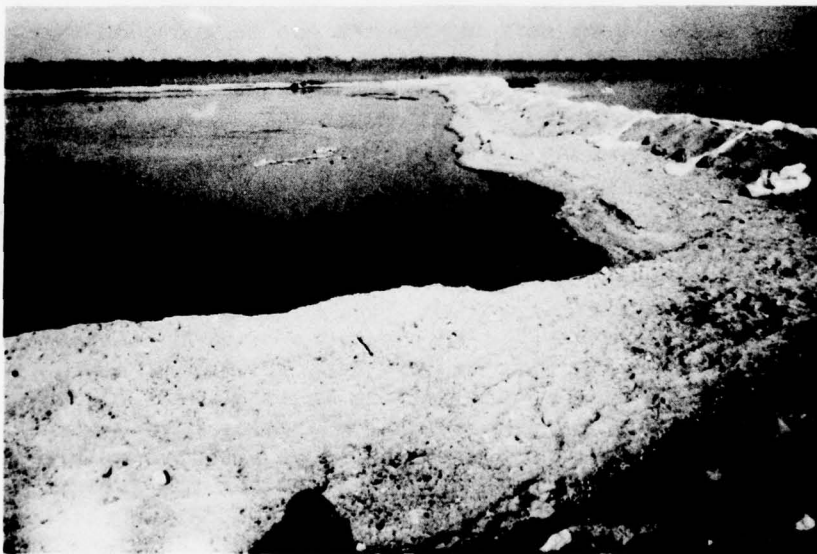
b. Sand dike after shaping to improve elevation
