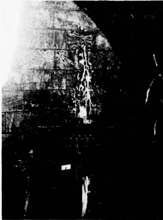
WATER DISCHARGING FROM 36 INCH GATE VALVE
