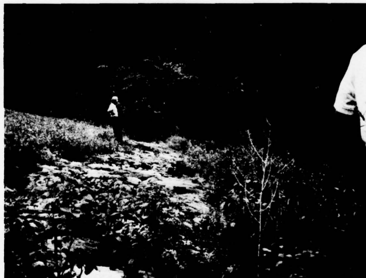
TOE OF DOWNSTREAM SLOPE
