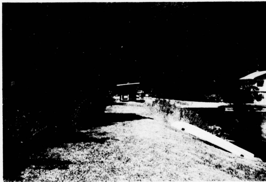
FIGURE 4. LEFT EMBANKMENT CREST
