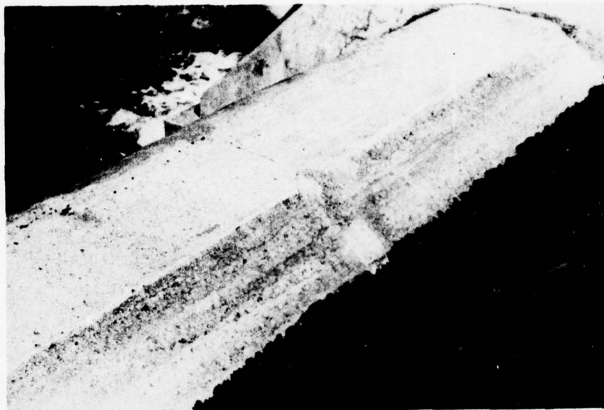
FIGURE 5. SPILLWAY CREST - PATCHED JOINT
