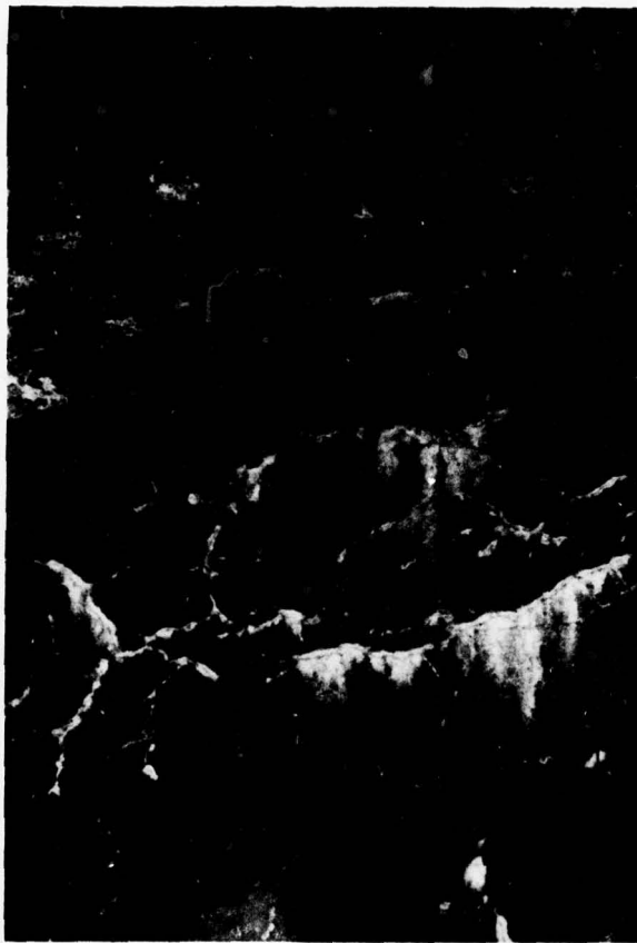
FIGURE 11. CRACKING AND SCALING OF MASSIVE CONCRETE BUTTRESS
