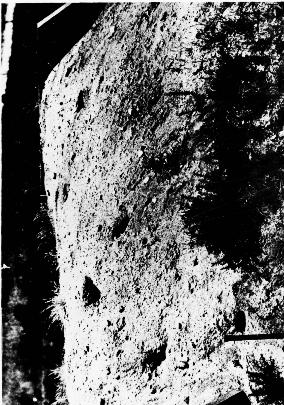
Figure 20. Ground Squirrel Burrows on an Ammunition Storage Bunker at Fort Hunter Liggett
