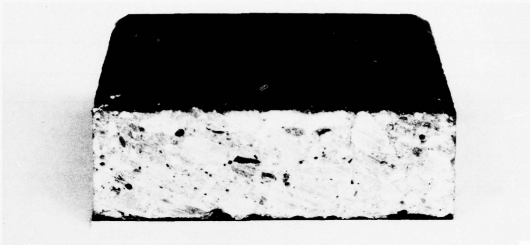
Figure 1. Sample of metallic finish concrete (DPS Masterplate).
