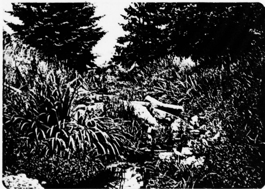
PLATE 6--Sample Site 2B 2 Upstream view of Riprap.
