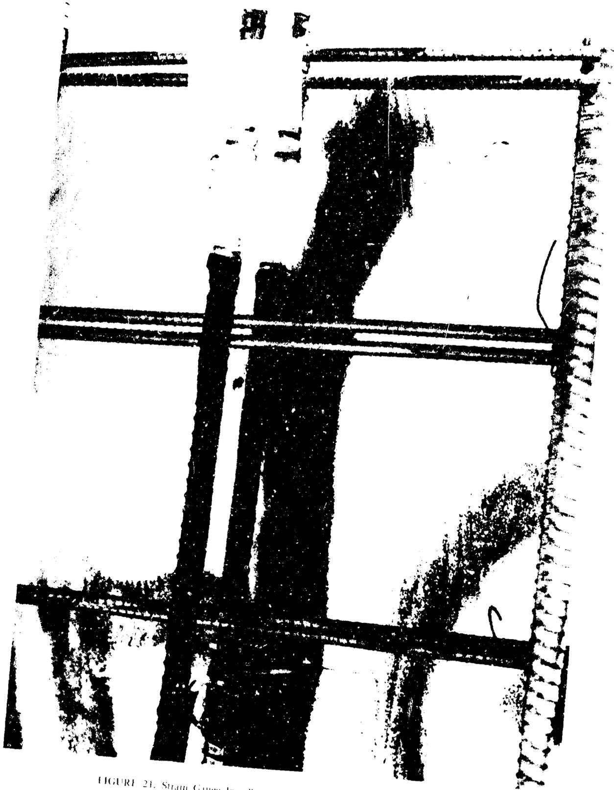
FIGURE 21. Strain Gauge Installation Prior to Concrete Pour, IRILOC Igloo.
